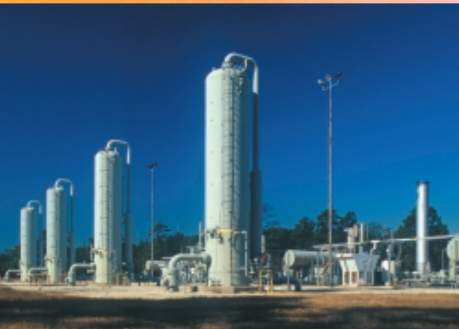
Bammel ▲ Gas Storage dehydration station
