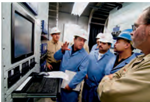
AEP Texas senior engineer Sam Hunt, left, observes while employees from Comisión Federal de Electricidad and an AEP contractor conduct final testing of a 4-MW NaS battery at Presidio, Texas. The installation enhances grid reliability along the Texas-Mexico border.
