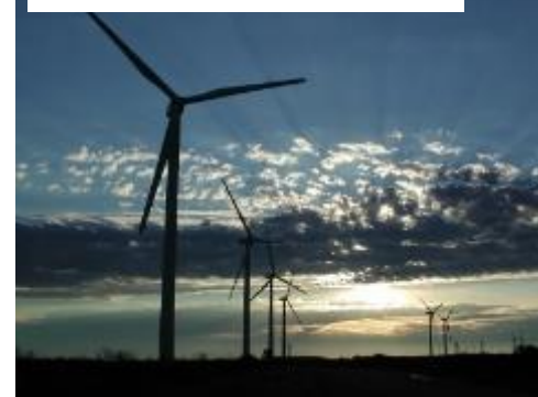
Trent Wind Farm (TX) – 154 MW
