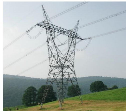
765 kV Transmission Line
