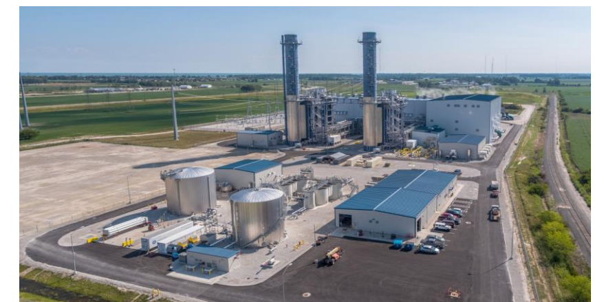
I&M filed for regulatory approval to acquire 870 MW Natural Gas Plant in Oregon, OH
