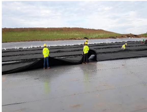
Photograph 1. Placing the Geocomposite Drainage Net.
