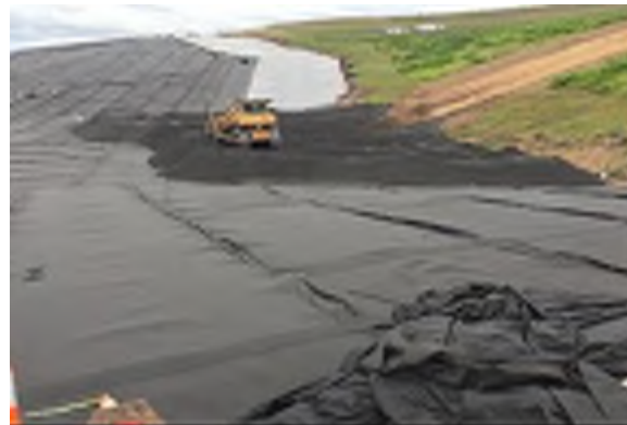
Photograph 5. Protective Cover being placed over the Geocomposite Drainage Net.
