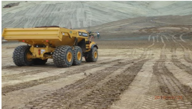
Photograph 10. Proof Rolling Subgrade
