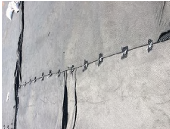
Photograph 4. Butt Seam Zip-Tied
