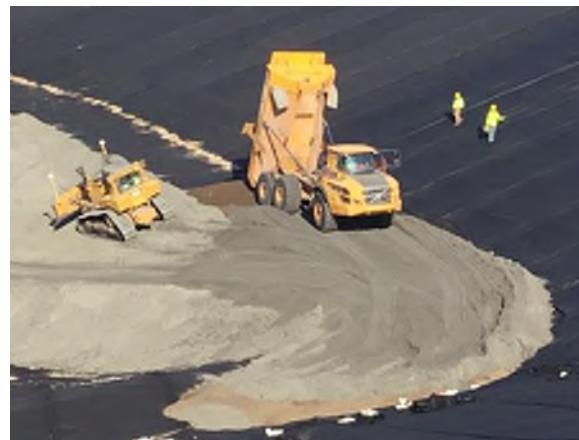
Photograph 8. No. 8 Stone Placement on B
