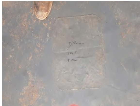
Photograph 10. Repair marked with date, time, initials of repairer
