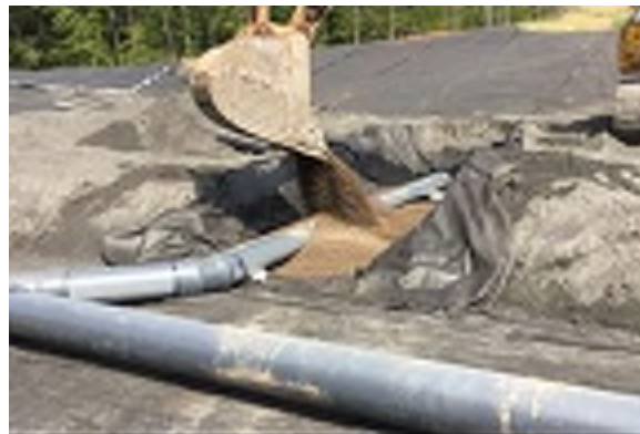
Photograph 6. Non-Calcareous Aggregate being placed around 12-inch Leachate Collection Pipe.
