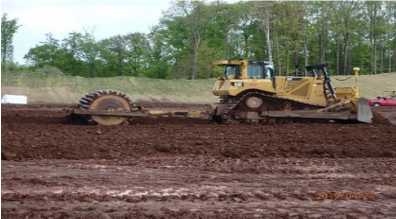
Photograph 5. Compaction
