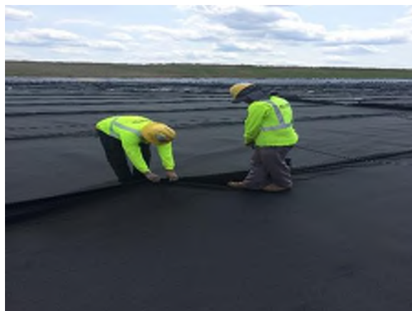
Photograph 3. Sewing Fabric Seam of the Geocomposite Drainage Net.
