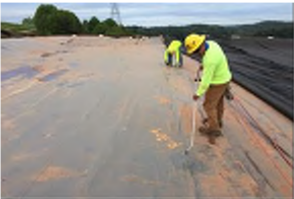
Photograph 9. Air Testing in progress
