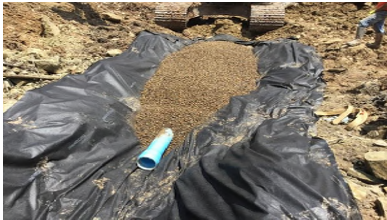
Photograph 7. Underdrain
