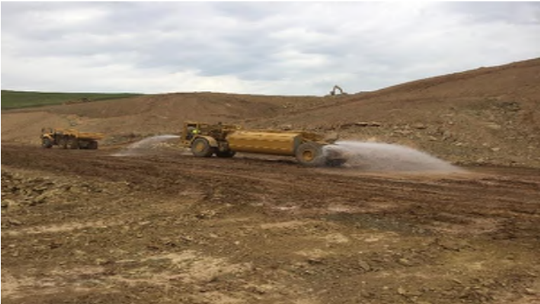
Photograph 5. Moisture Addition
