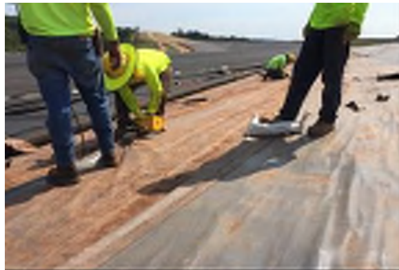
Photograph 11. Seaming in progress
