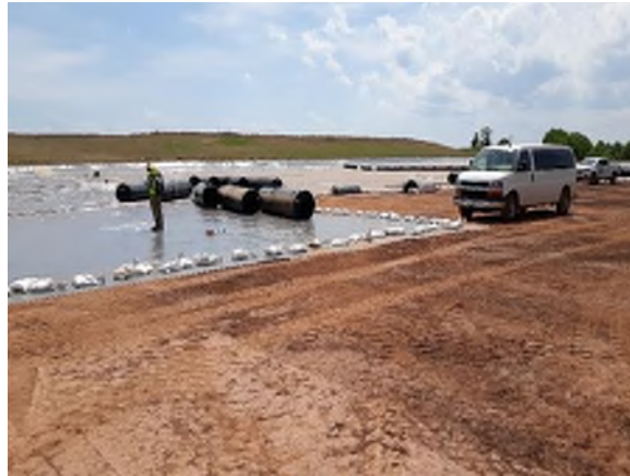
Photograph 1. PVC Deployed on West flat area
