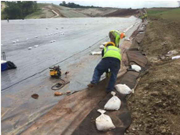
Photograph 4. Preparing to seam
