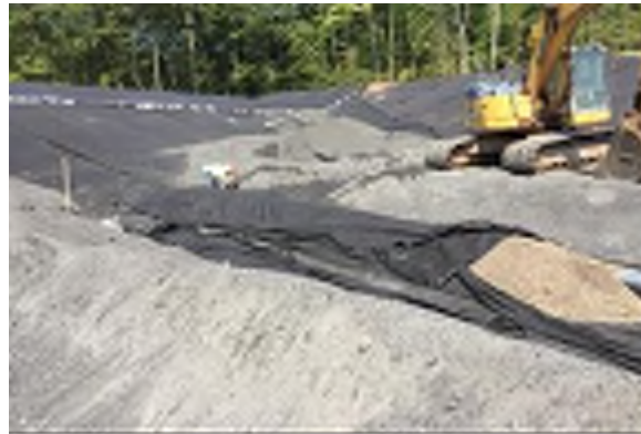
Photograph 7. Leachate Collection Pipe and Aggregate wrapped with 6-oz Geotextile
