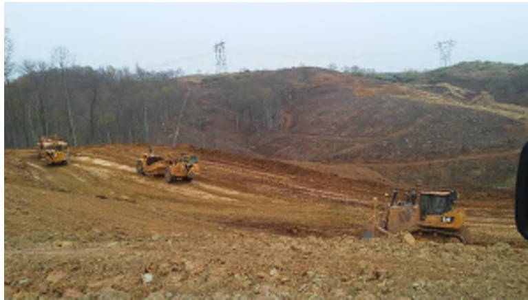
Photograph 1. Topsoil Removal
