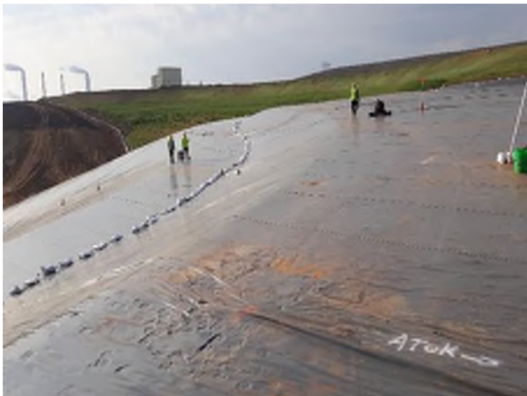
Photograph 8. Air Testing denoted with "ATOK"
