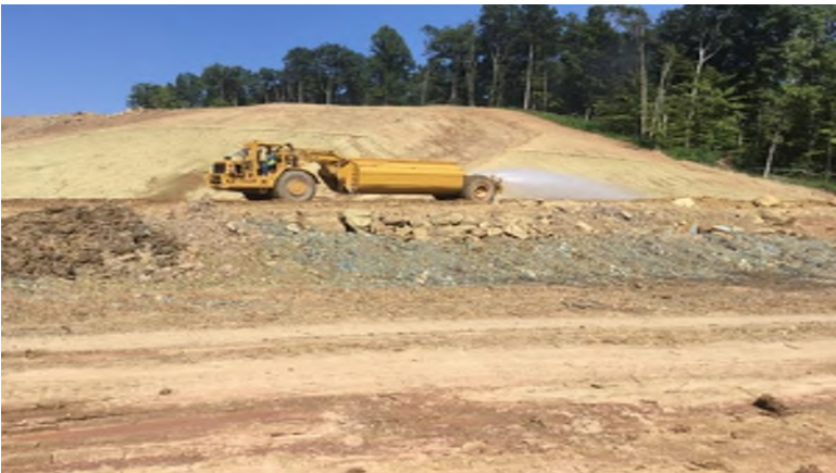
Photograph 6. Moisture Addition
