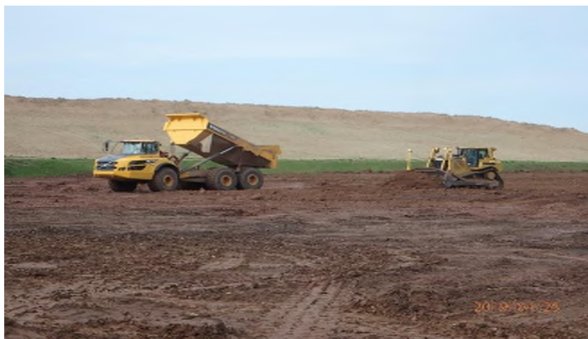
Photograph 3. Clay Placement
