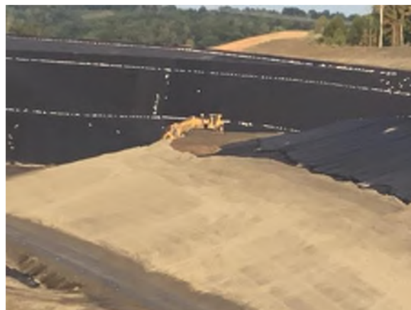
Photograph 9. Lower Slope covered with Protective Cover - East Area
