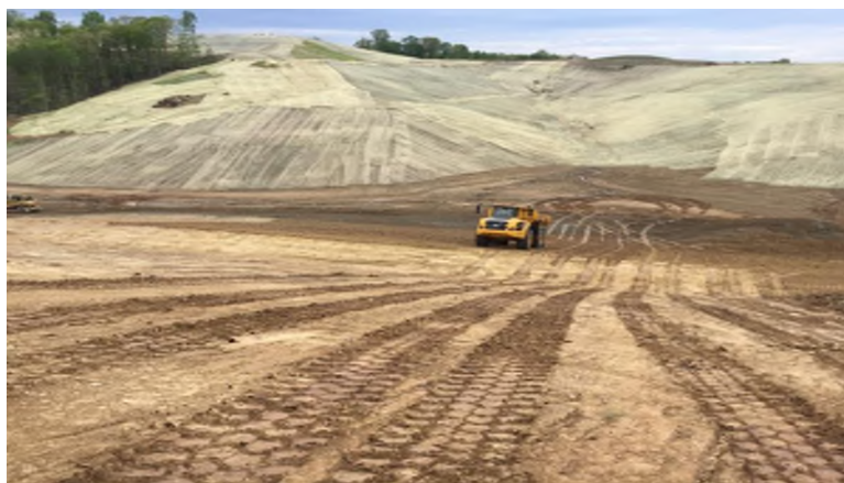
Photograph 9. Proof Rolling Subgrade
