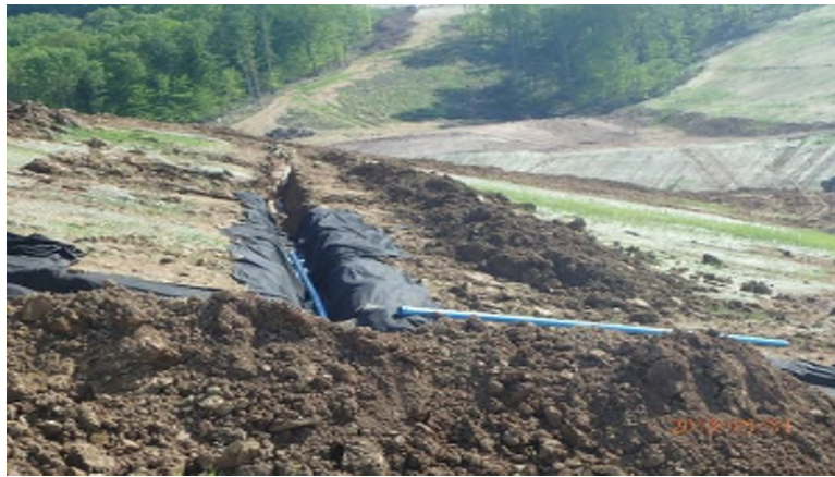
Photograph 8. Underdrain
