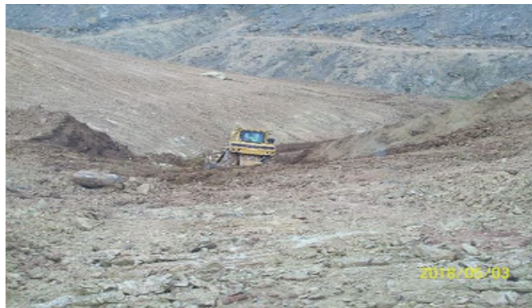
Photograph 2. Topsoil Removal
