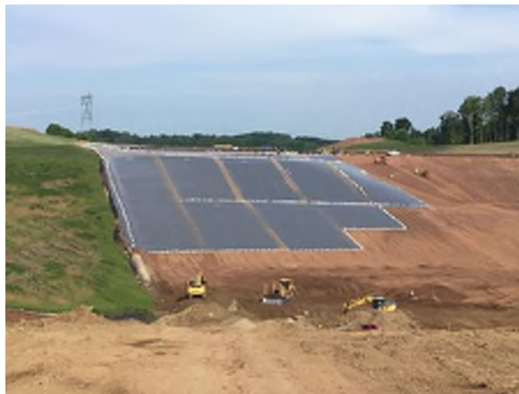
Photograph 3. West slope covered with PVC
