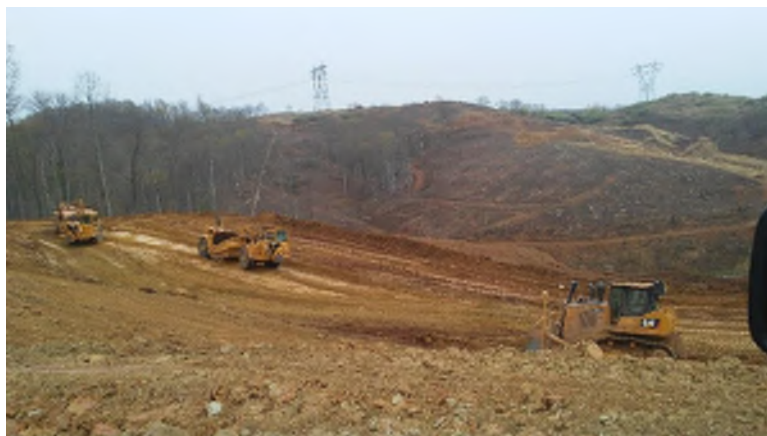
Photograph 3. Excavation with Construction Equipment
