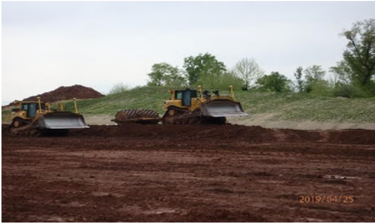
Photograph 6. Compaction
