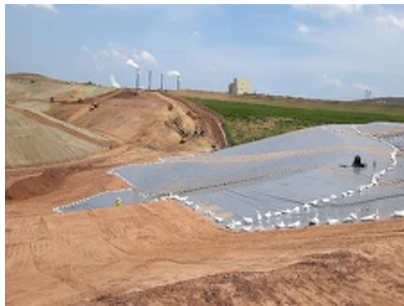
Photograph 2. West area slope covered with PVC
