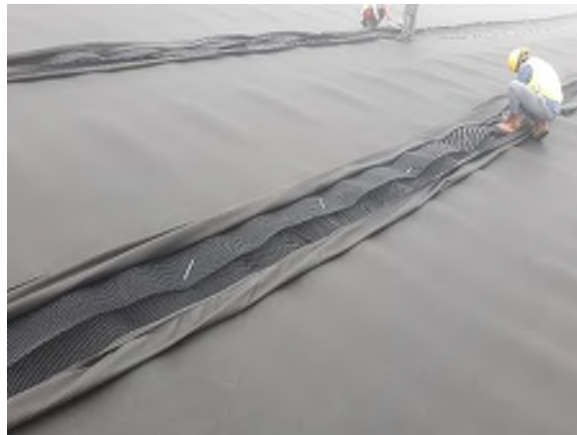
Photograph 2. Zip-tying Geocomposite Drainage Net.
