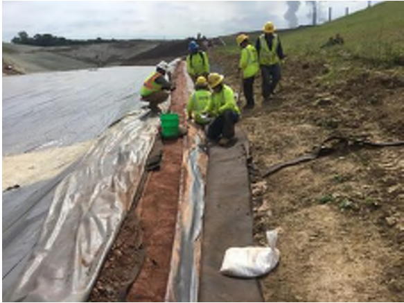
Photograph 5. Cleaning prior to seaming
