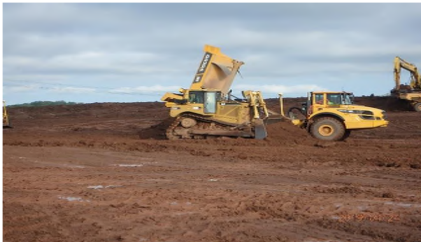
Photograph 2. Clay Placement
