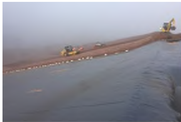
Photograph 12. Rock Hounding, Smooth drumming CCL
