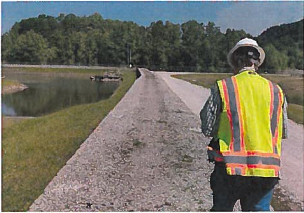
Photo 1 – Typical view of block wall and inboard slope showing good conditions.
