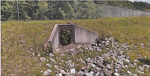
Photo 7 – Typical view of the reclaim' s pond 36 inch diameter HDPE overflow pipe showing good conditions with no obstructions to flow and no visible erosion.
