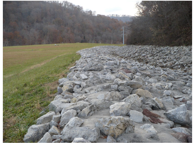
Photo #6 – Pond 1A diversion ditch
