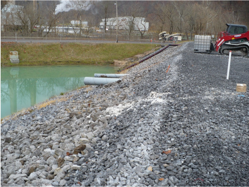
Photo #17 – reclaim pond interior slopes
