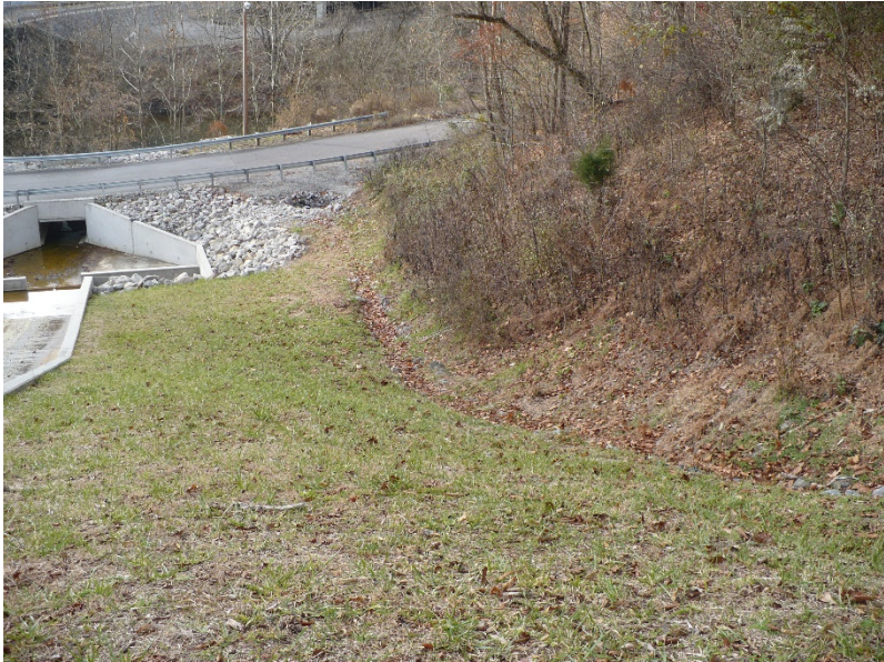
Photo #9 – right abutment, 25-ft clear zone
