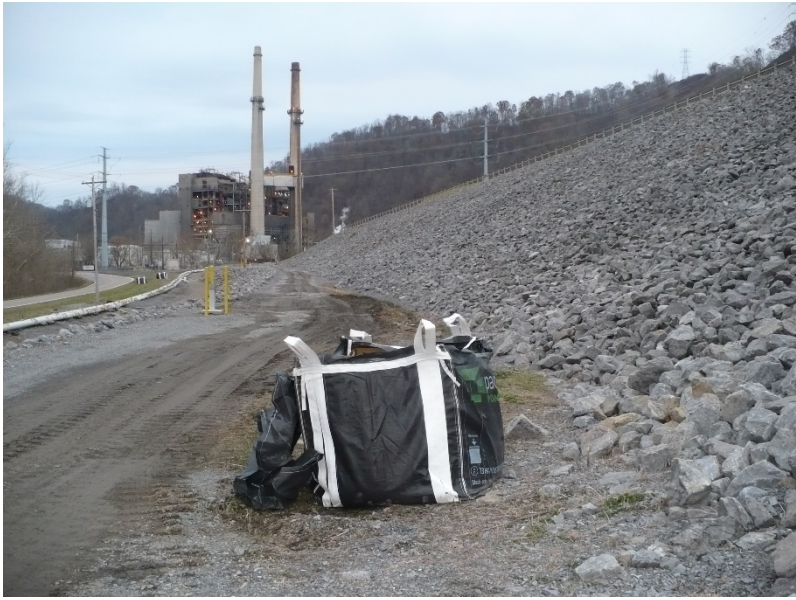
Photo #3 – exterior slope of Pond 1A
