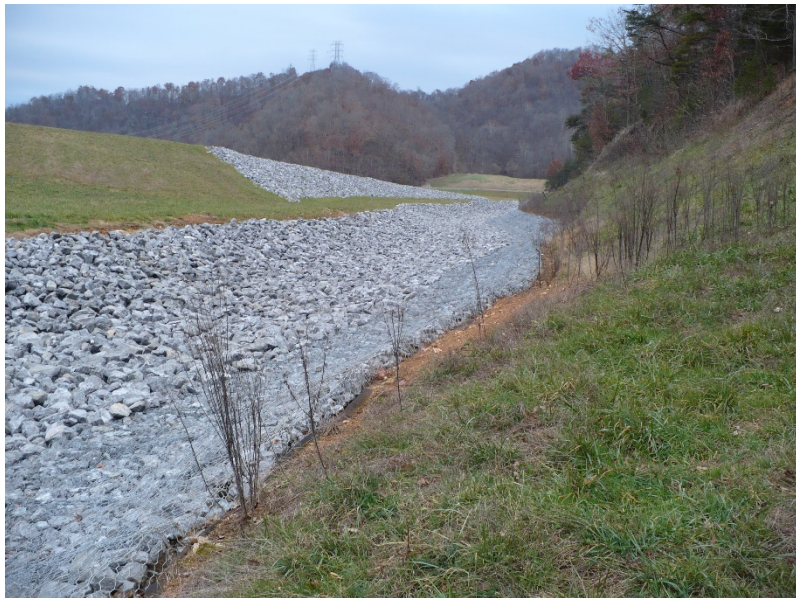
Photo #15 – Pond 1B diversion ditch
