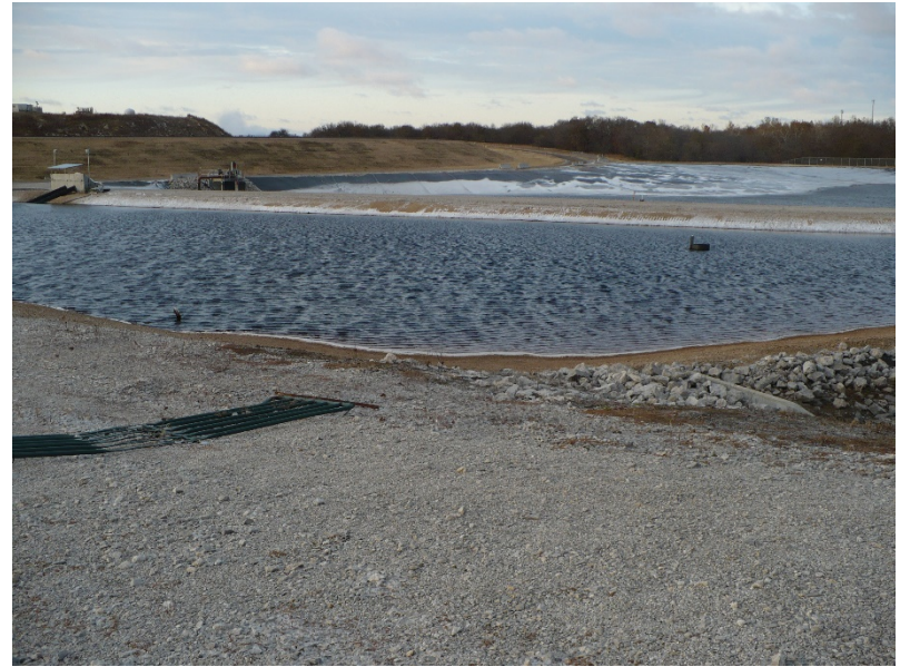
Photo #6 – Leachate collection pond – almost full
