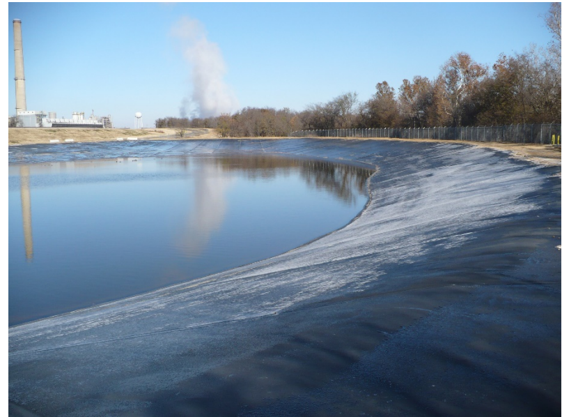
Photo #8 – Interior slope of non-contact water pond (Basin C)
