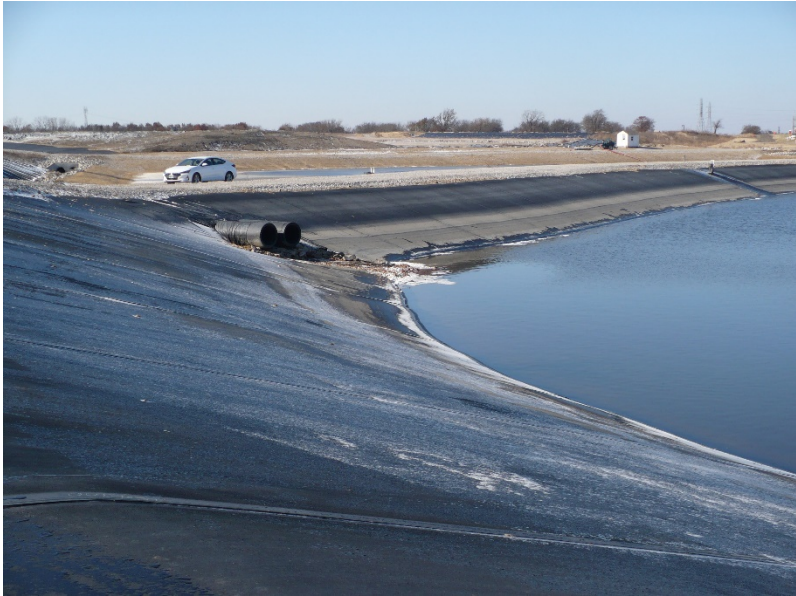
Photo #9 – outlet of south non-contact water culverts into Basin C
