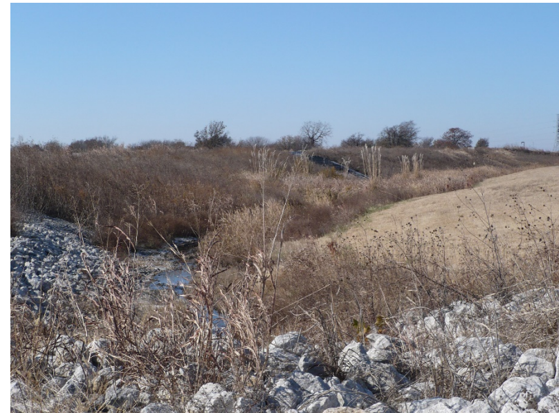
Photo #4 – exterior slope North containment berm-looking west
