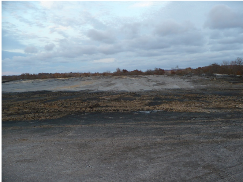
Photo #1 – active disposal Cell 2
