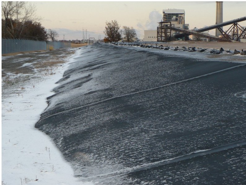
Photo #3 – geomembrane cover of west slope
