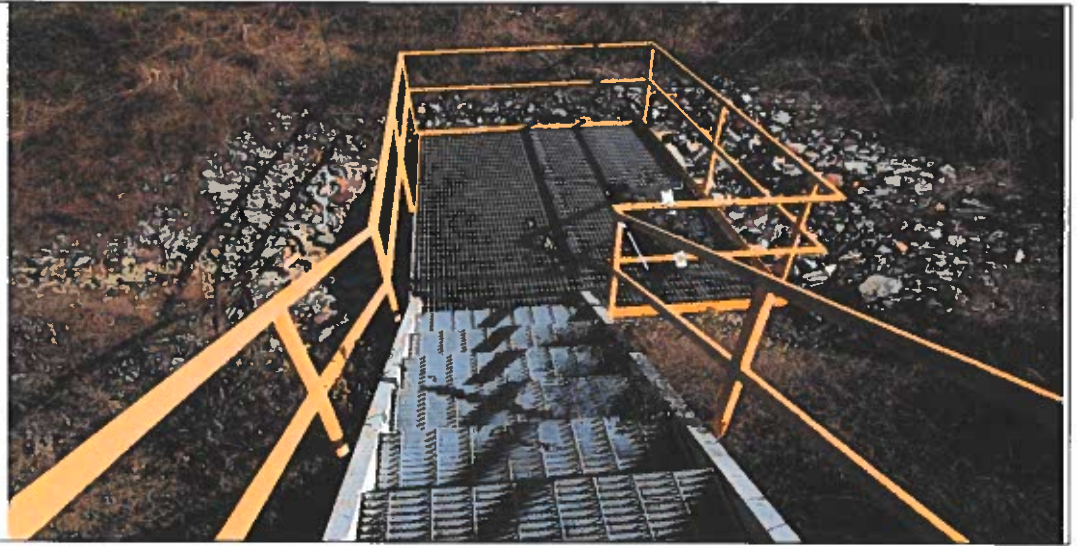
Photo #19 The overflow pipe discharge structure.
