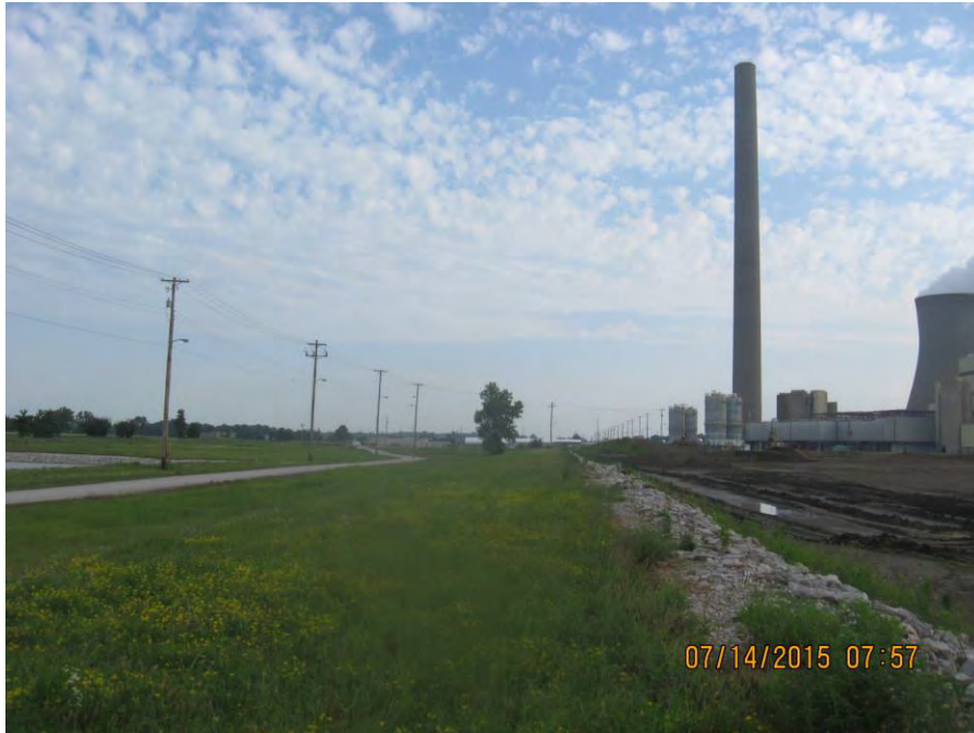
Photo 5: West Bottom Ash Pond, west dike: crest and interior slope (facing north).
