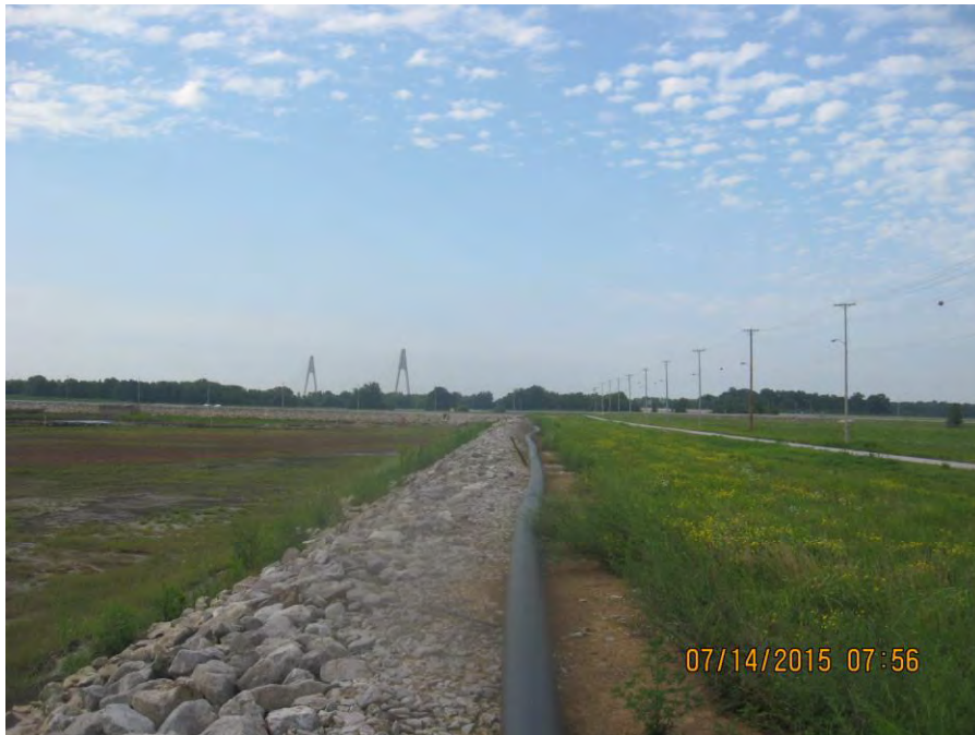
Photo 4: West Bottom Ash Pond, west dike: crest and interior slope (facing south).
