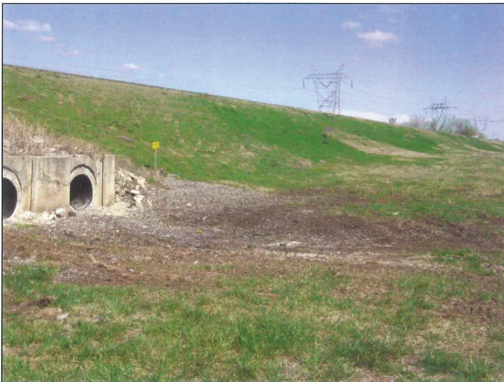
Figure 6 – Downstream Basin with Culverts
