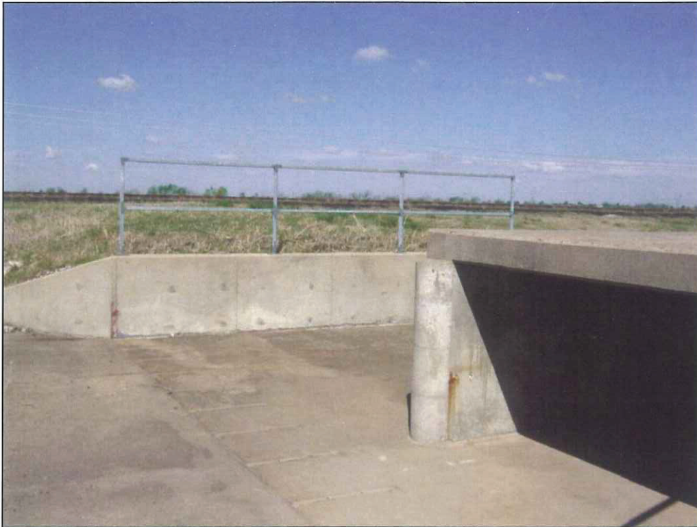
Figure 5 – Bottom Ash Pond Spillway
