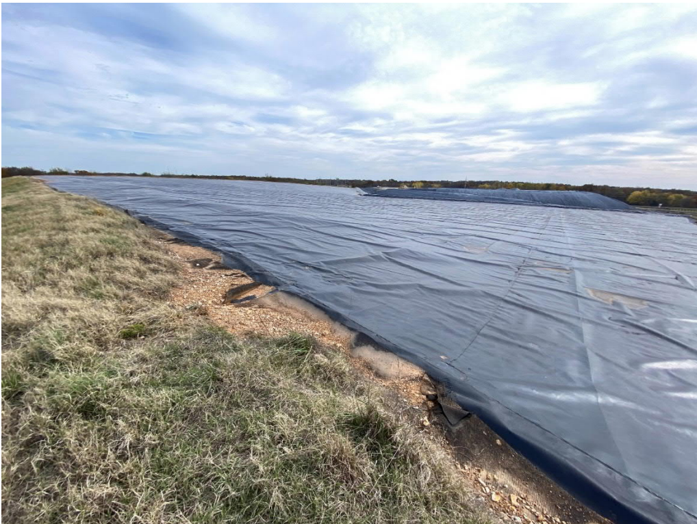
6. Exposed geomembrane of the inactive area looking southeast from the northwest corner.
