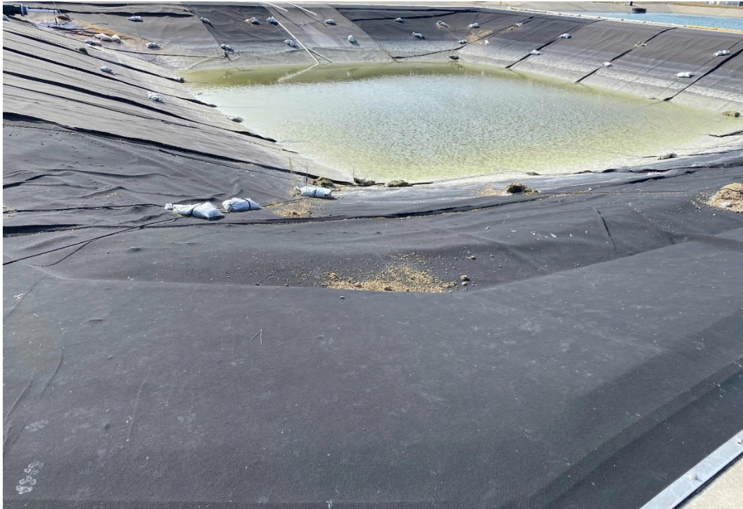
9. Leachate Collection Pond.
