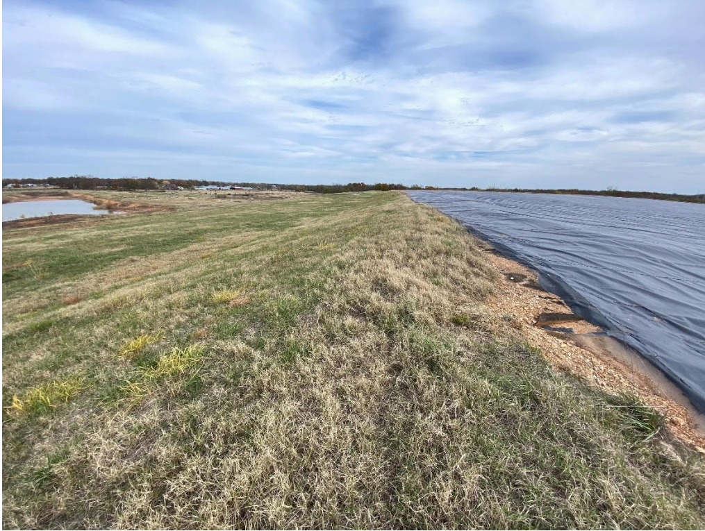
19. North side final cover looking east.
