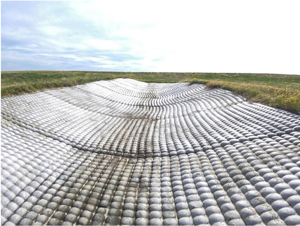
7. Fabriform letdown on the north closed area of the landfill.
