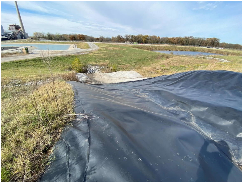
4. Inactive area letdown on the southwest corner of the inactive area.
