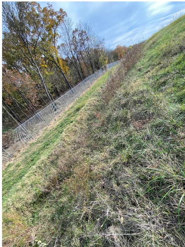
16. Stormwater ditch on the east side of the landfill.
