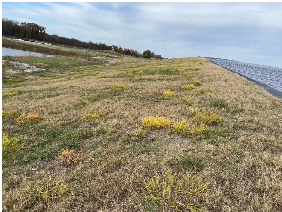
18. West side final cover slope looking north.
