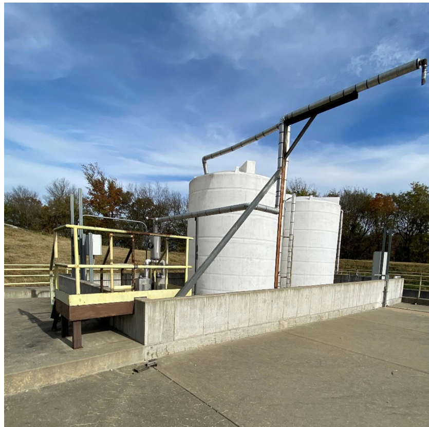
10. Inactive leachate sump on the southeast corner of the landfill.
