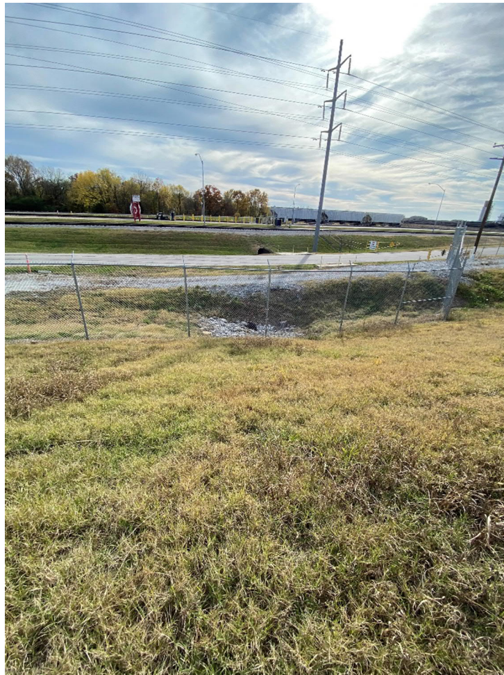
17. Stormwater culvert on the south side of the landfill.
