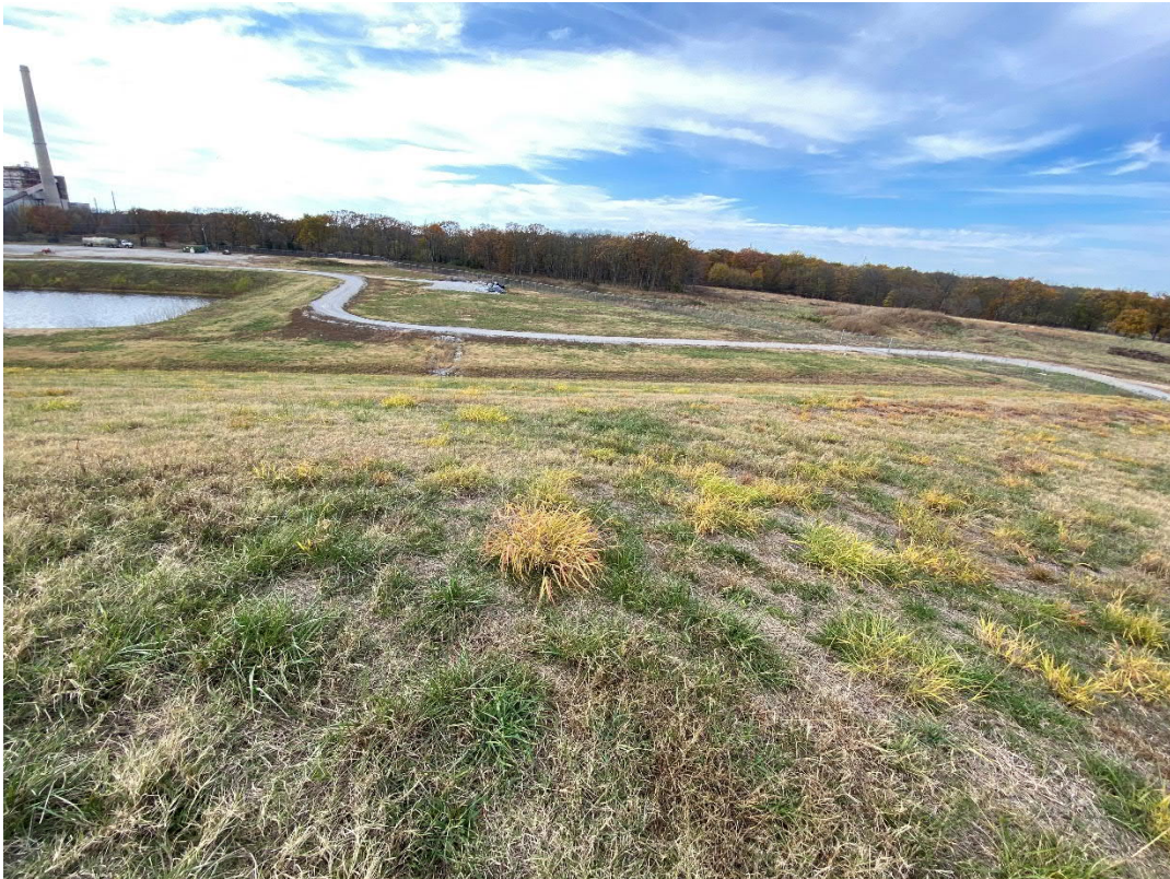
14. Stormwater ditch on the west side of the landfill.
