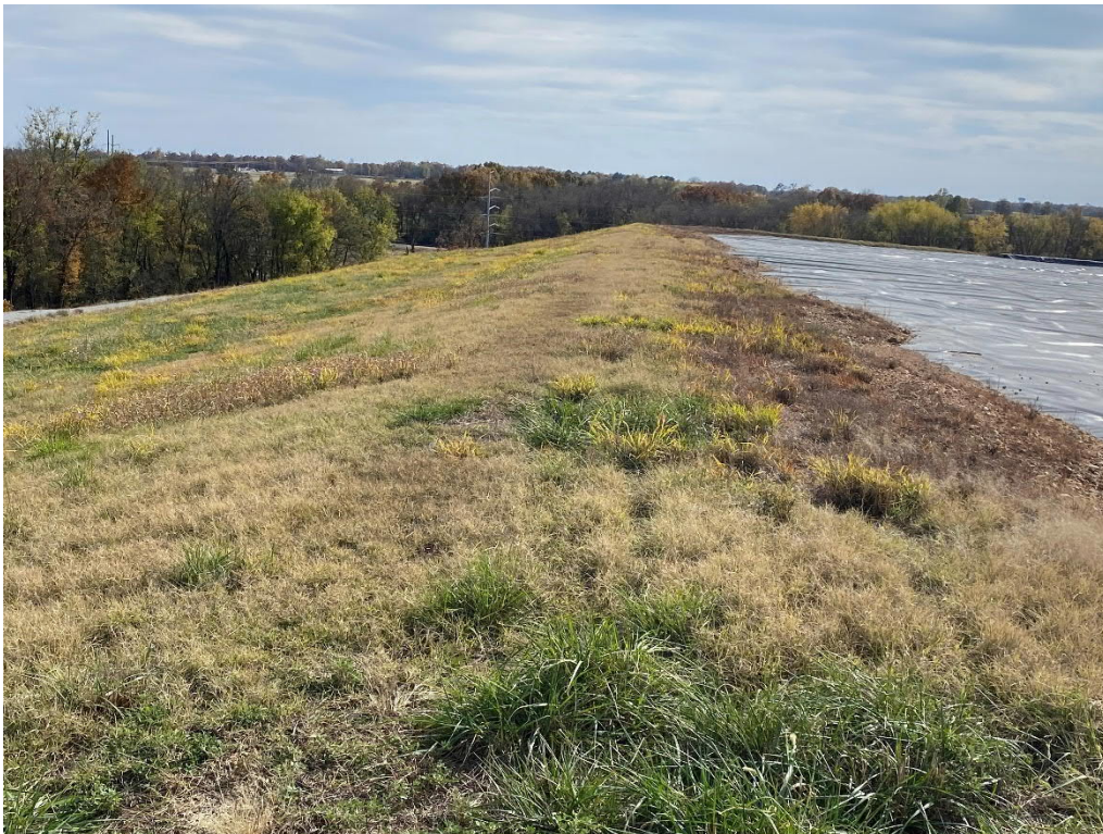
20. East side final cover looking south.
