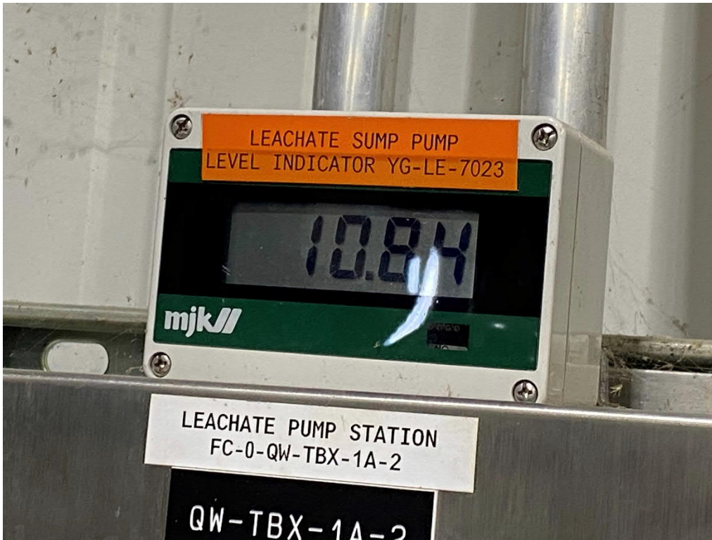
11. Leachate pond sump level indicator.
