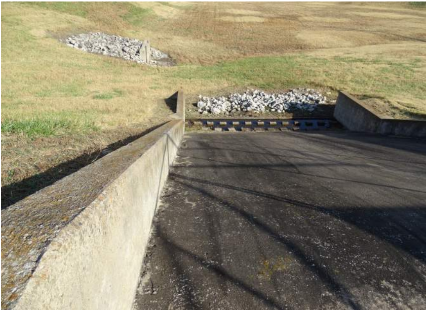
Photo #5 - Spillway chute looking north
