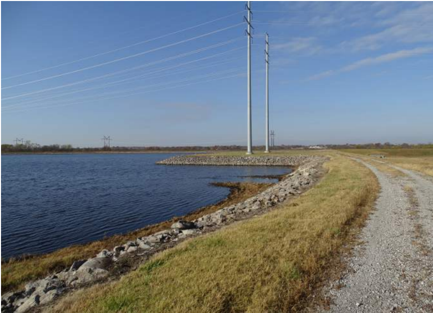
Photo #3 - Upstream slope of north dike, looking west
