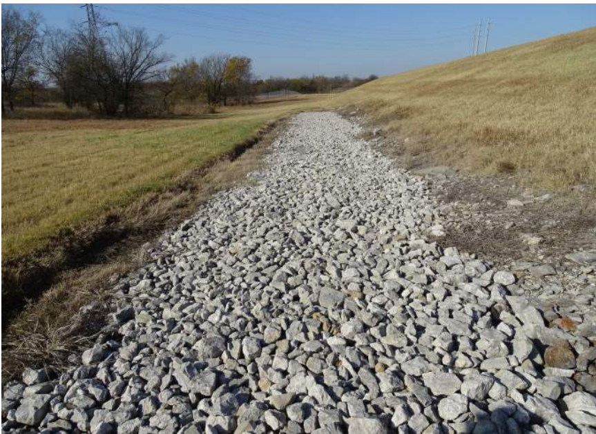
Photo #11 - South downstream embankment looking west
