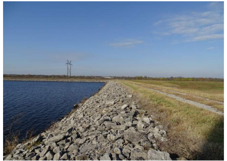
Photo #2 - Upstream slope of north dike, looking west
