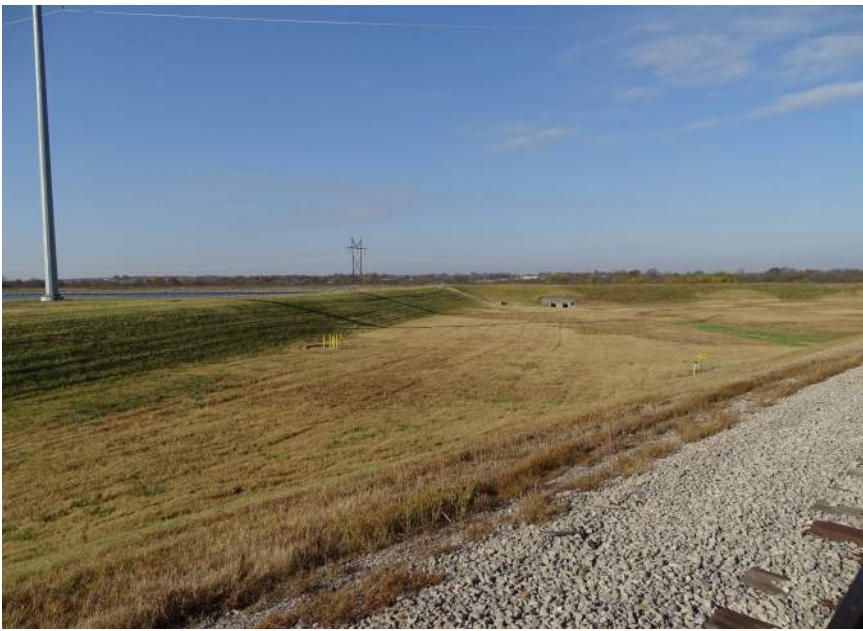
Photo #1 - Exterior slope north dike, looking west
