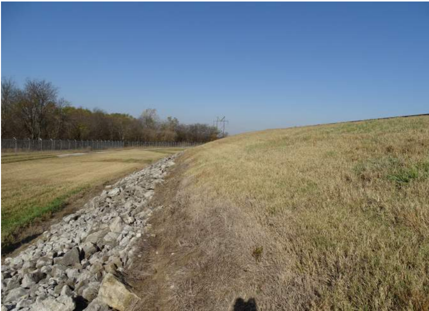
Photo #7 - Downstream slope of west dike, looking northeast
