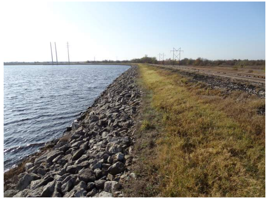
Photo #6 - Upstream slope of west embankment, looking south
