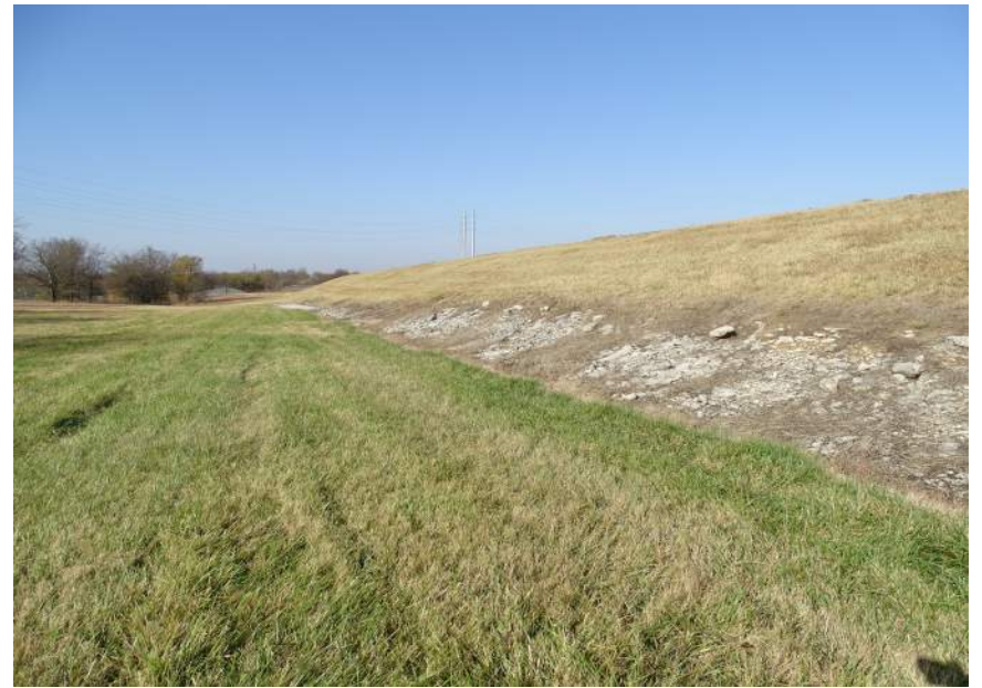
Photo #10 - South downstream embankment looking west
