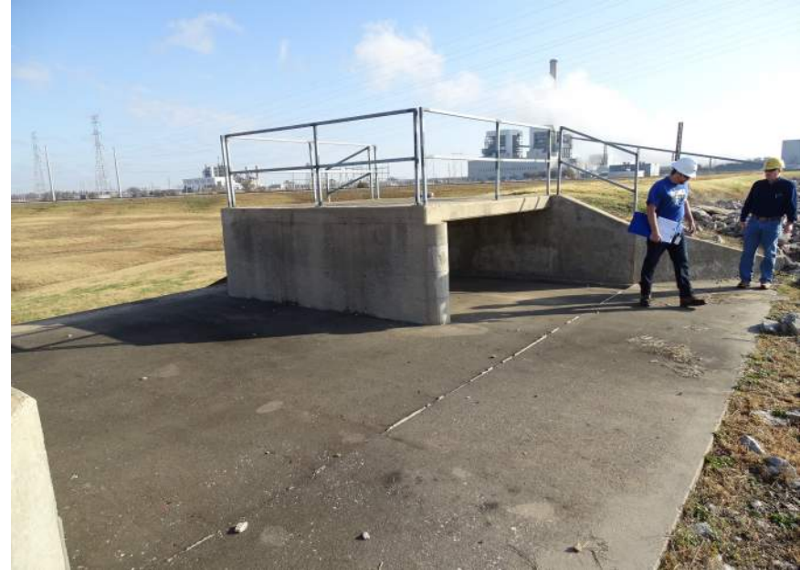
Photo #4 - Auxiliary spillway
