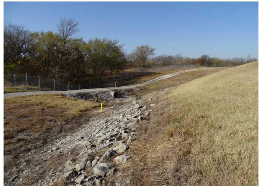
Photo #12 - Drainage culvert at the bend between south and west embankment
