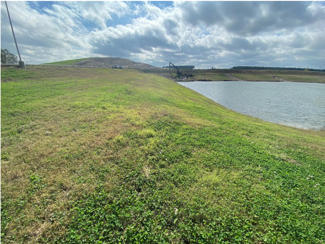
7. East slope of the leachate collection pond facing south.
