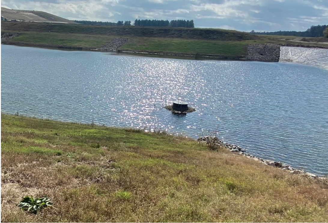
6. Leachate pond inlet structure on the northwest corner of the pond.
