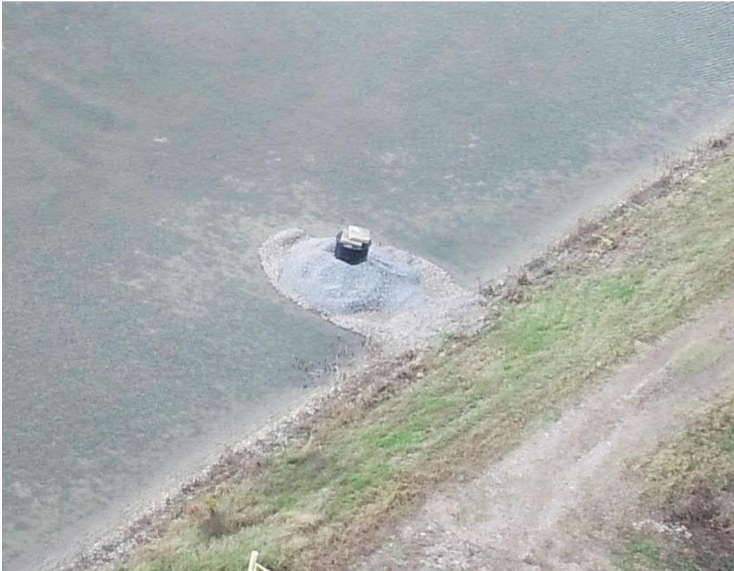
16. The inlet of the overflow discharge structure for the stormwater pond.
