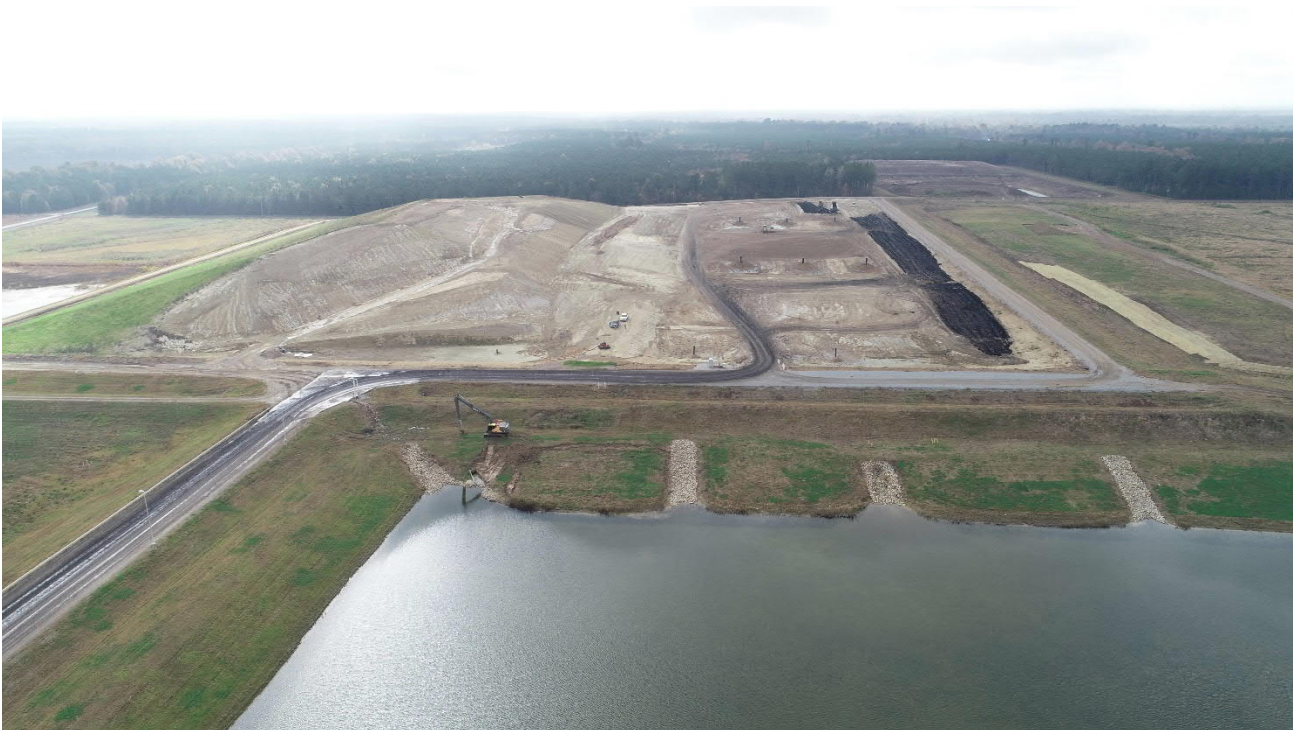
11. The north side of Cells 1 & 2 looking to the south.
