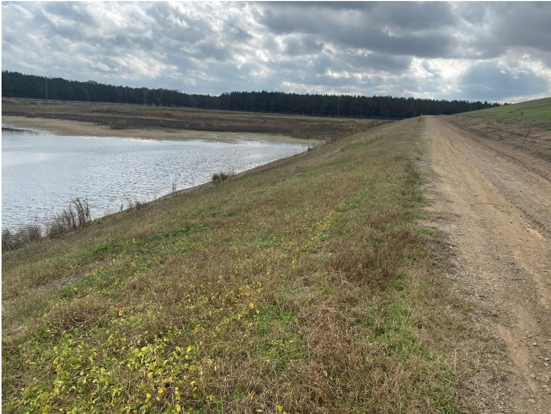
8. The east side berm that is between Cell 1 and the stormwater pond.
