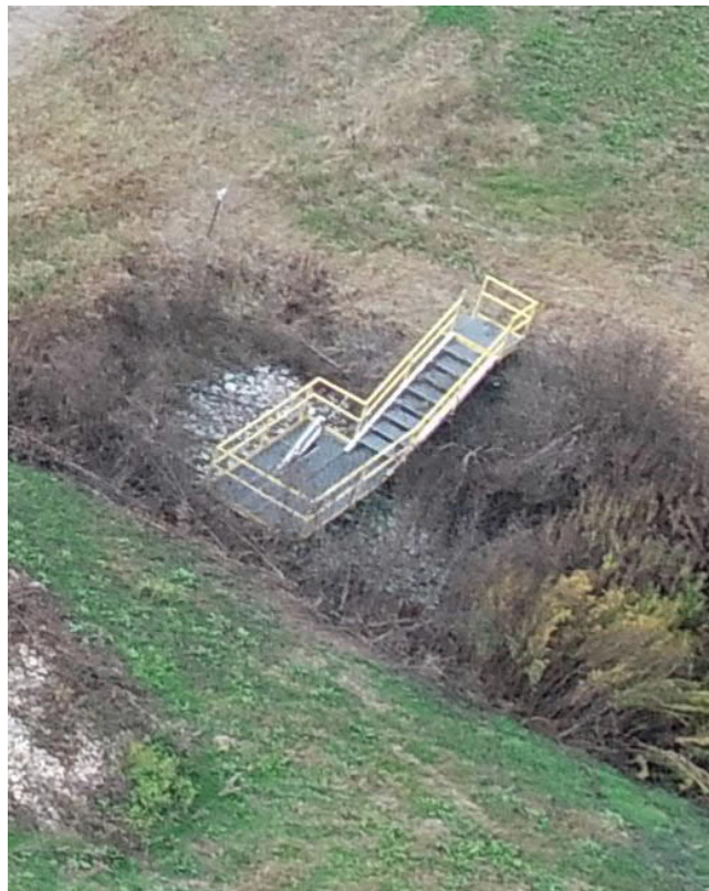
17. The overflow pipe discharge structure for the stormwater pond.
