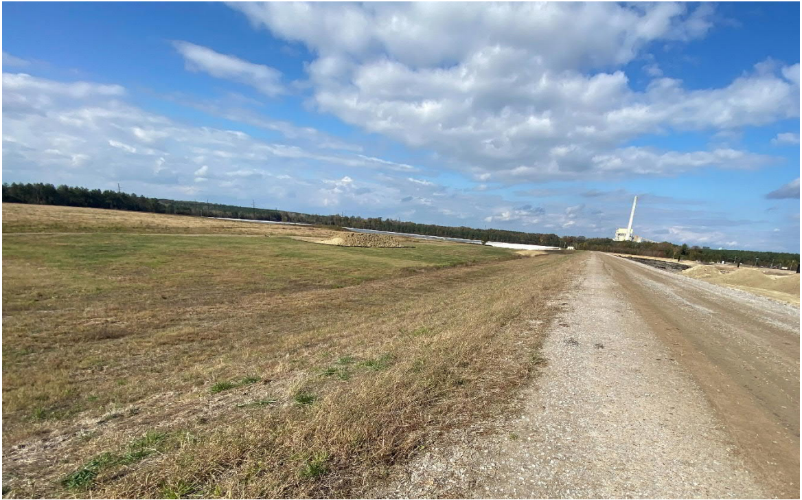
12. Road and berm on the west side of Cell 2.
