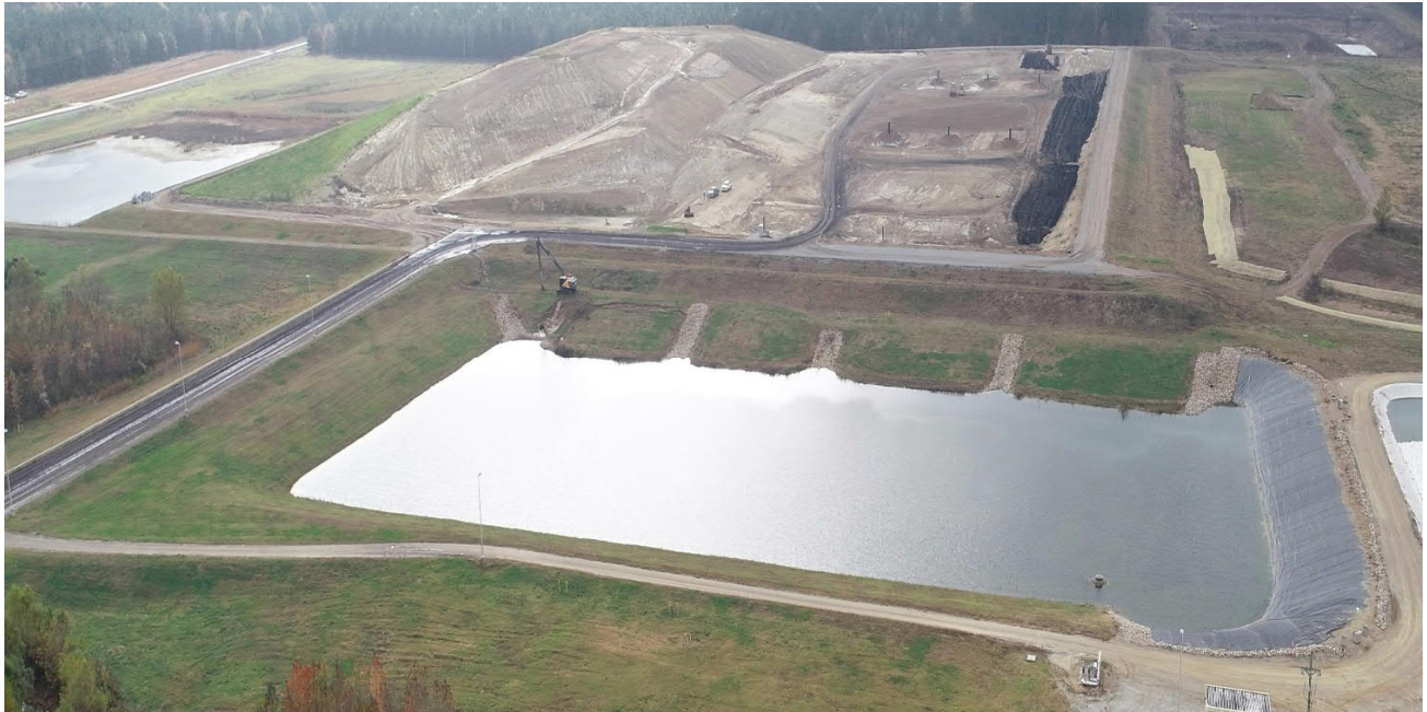
1. Leachate Collection Pond looking from the north side.
