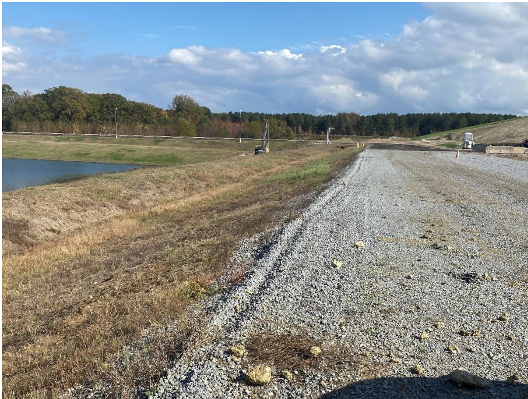
13. Road, berm and stormwater ditch between Cell 2 and the leachate collection pond.
