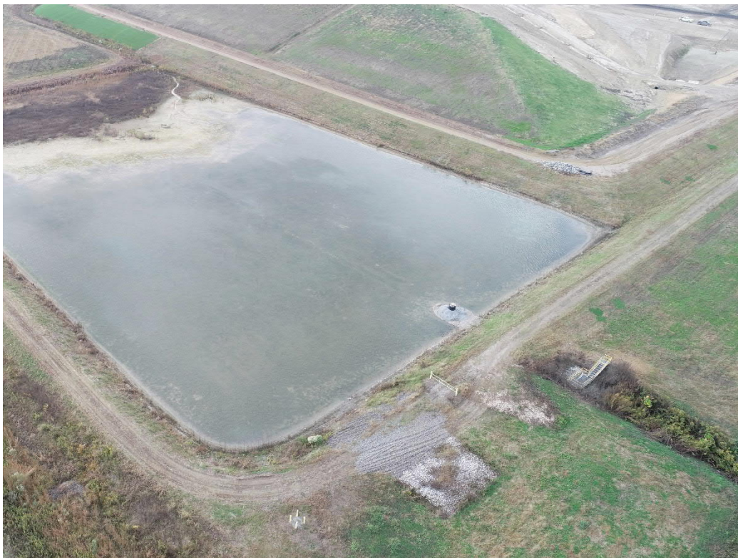
15. An overall view of the stormwater pond.
