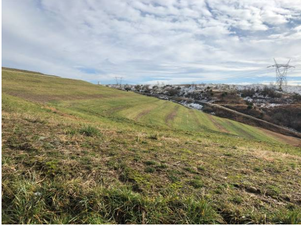
Photograph 5: View of the final vegetated cap on the south face of Sequence 3.
