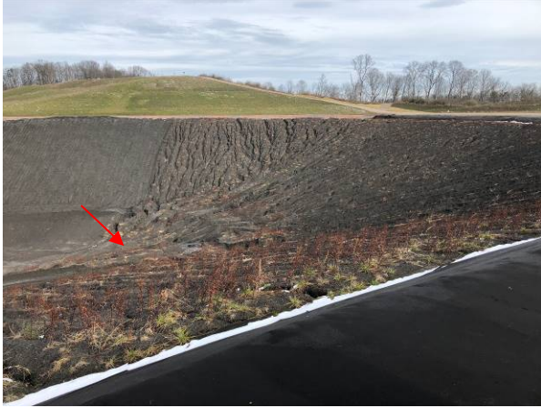
Photograph 1: View of the eastern bowl of Sequence 4. The location of the groundwater bubbles under the liner are noted by the red arrow.
