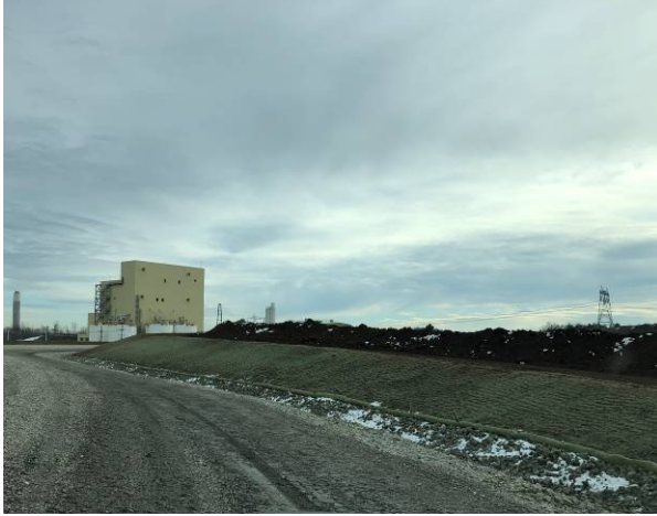
Photograph 14: View of the temporary soil cover on the north side of Sequence 1. This area had been recently hydro seeded.
