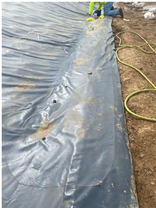
Photo 3: Applying chemical adhesive patch.
