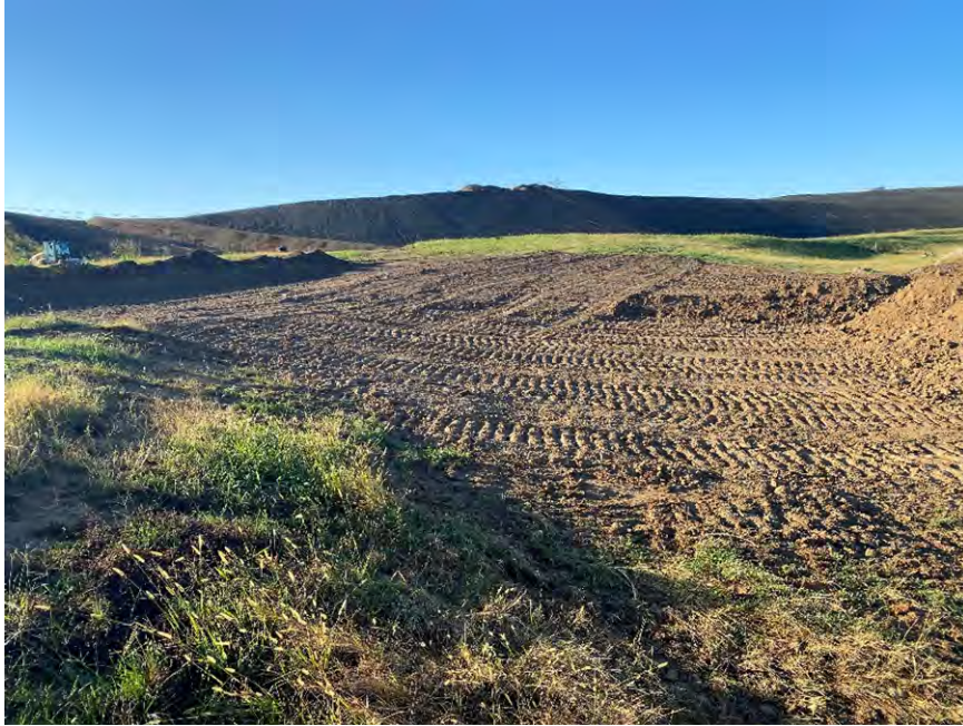
Photo 1: Clay backfill placed on berm on prior day.
