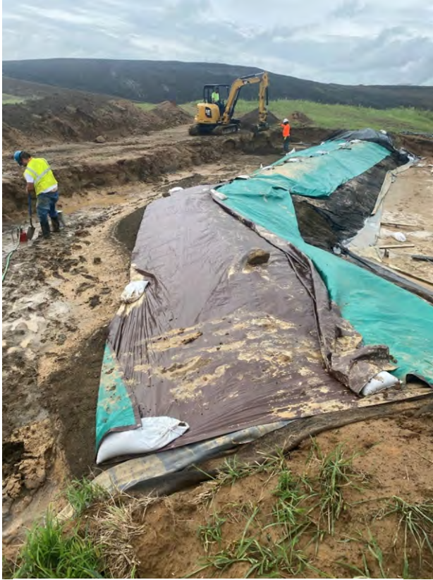
Photo 1: Removal of saturated materials behind intermediate berm (landfill side).
