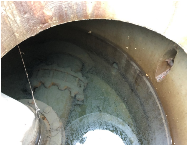
Photograph 4: View inside Manhole #13 before pumping out the standing (clean water).
