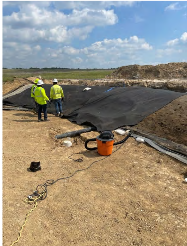
Photo 2: Looking north CCS has begun covering up the berm with geotextile.
