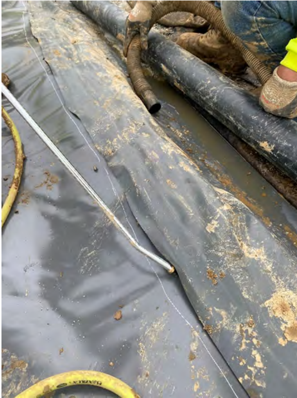
Photo 3: Air lance testing wedge weld seam at floor.
