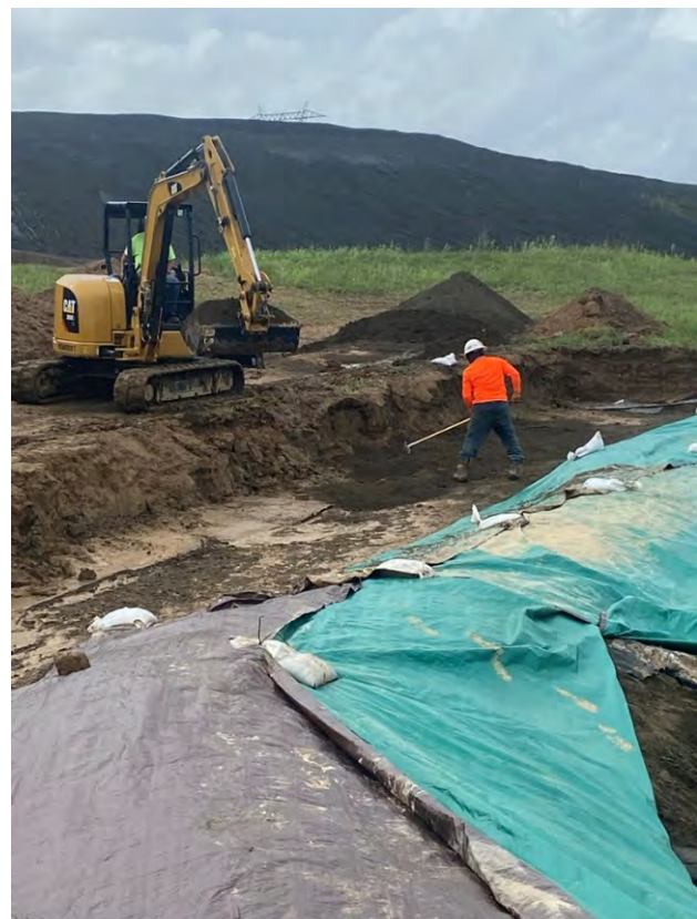
Photo 2: Placement of bottom ash behind intermediate berm (on landfill side).
