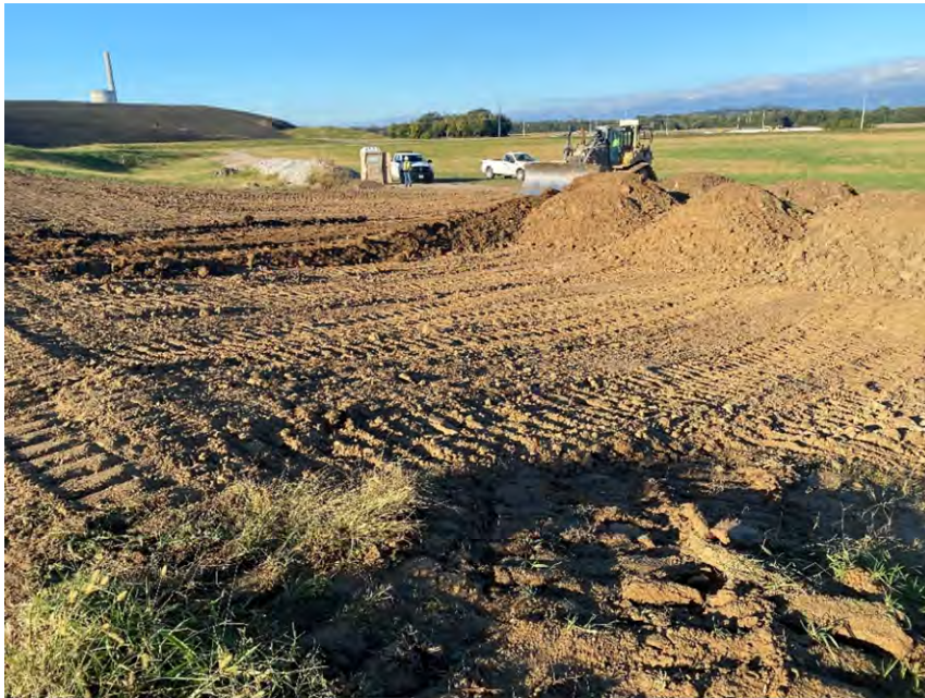
Photo 2: Topsoil stockpiled and ready for placement.
