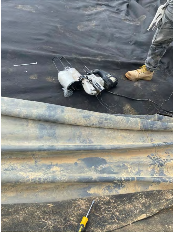
Photo 1: Sewing machine being used to stitch the geotextile panels together.
