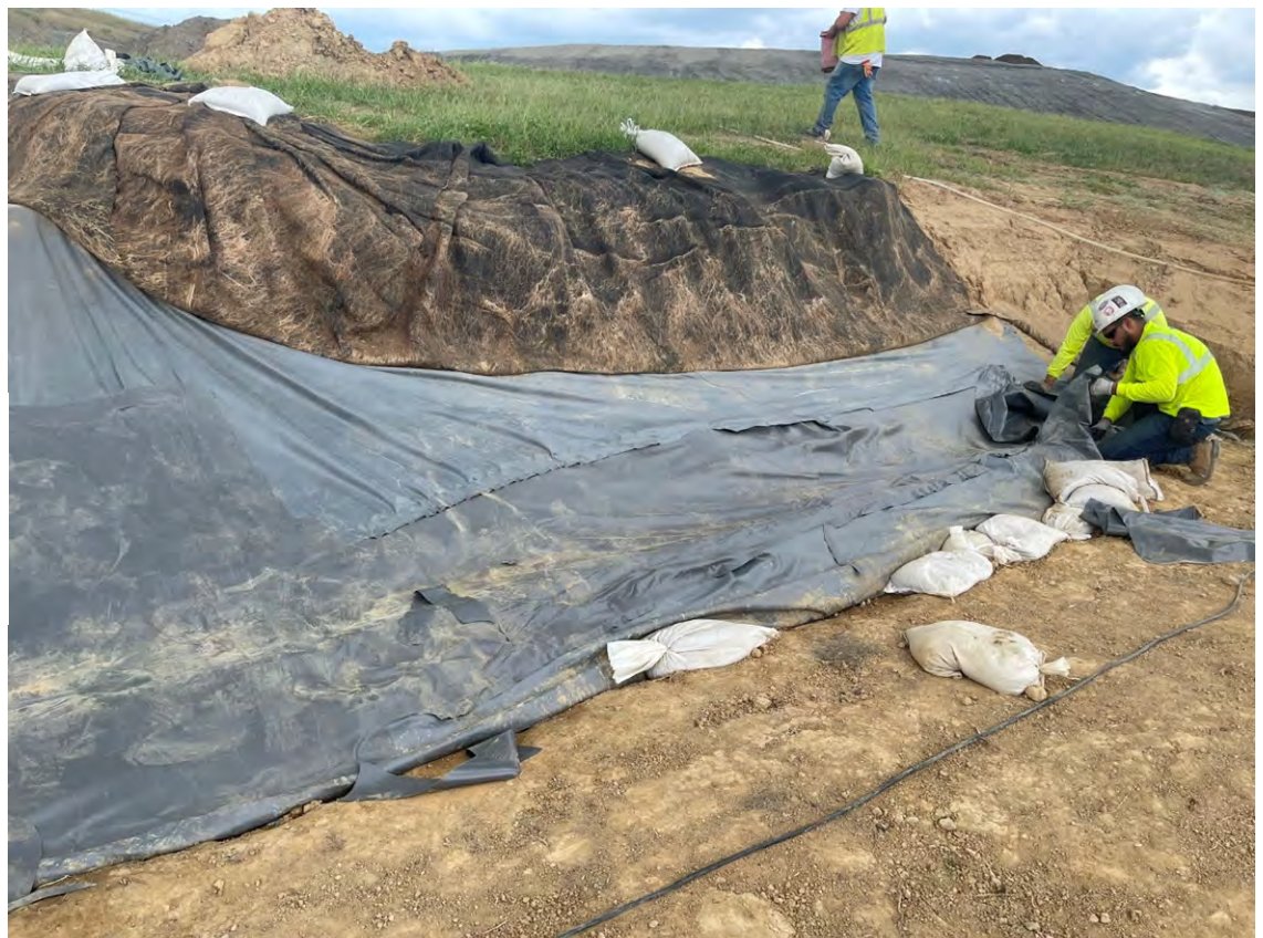
Photo 2: Looking at the south end tie-in points.
