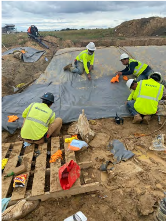
Photo 2: Preparing area to apply adhesive chemical patch.
