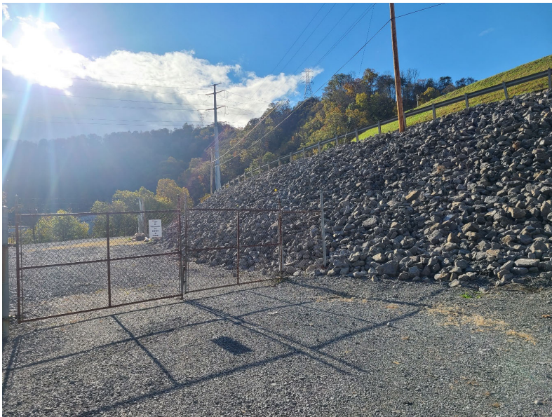
Photo #3 – exterior slope of Pond 1A
