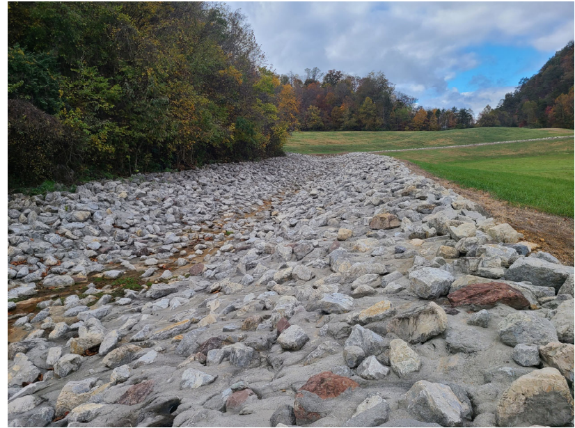
Photo #6 – Pond 1A diversion ditch
