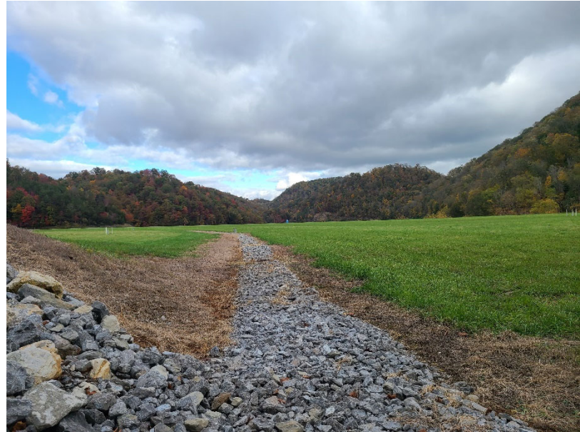
Photo #14 – drainage swale into Pond 1A diversion channel
