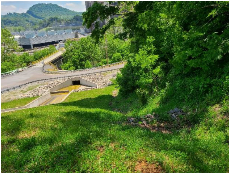
Photo #9 – right abutment, 25-ft clear zone
