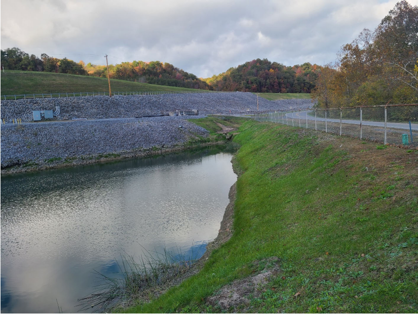
Photo #17 – reclaim pond interior slopes
