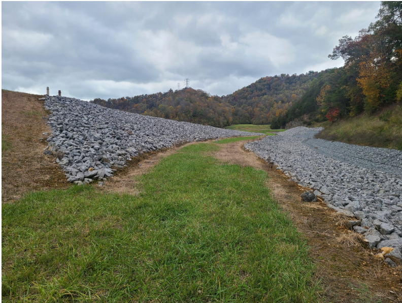
Photo #15 – Pond 1B diversion ditch
