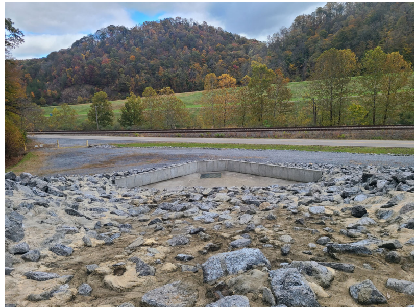
Photo #14 – drainage swale into Pond 1A diversion channel
