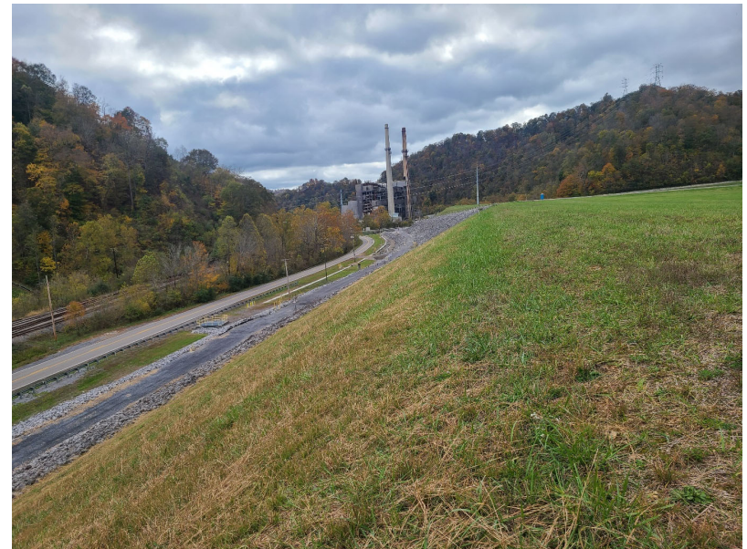
Photo #4 – grass cover on slopes of Pond 1B, above riprap
