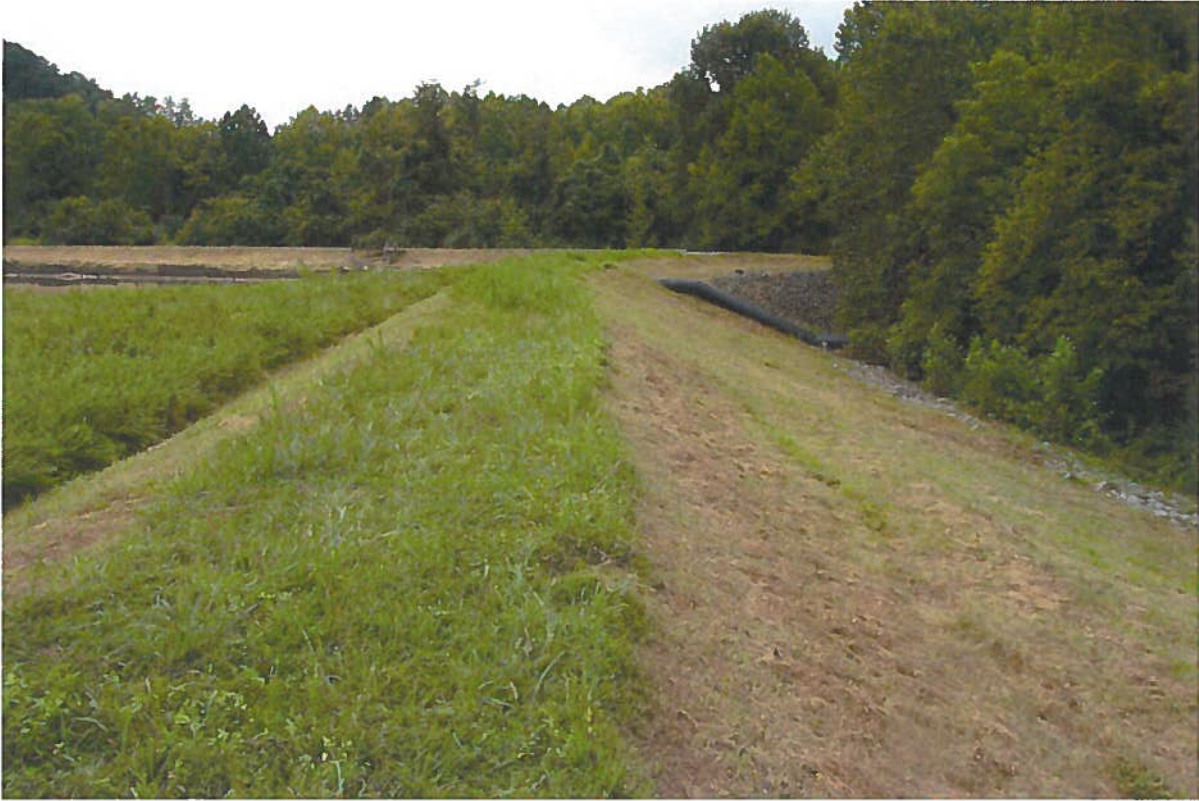
Photograph 1. Pond 1B Spillway Pipe and Downstream Slope
