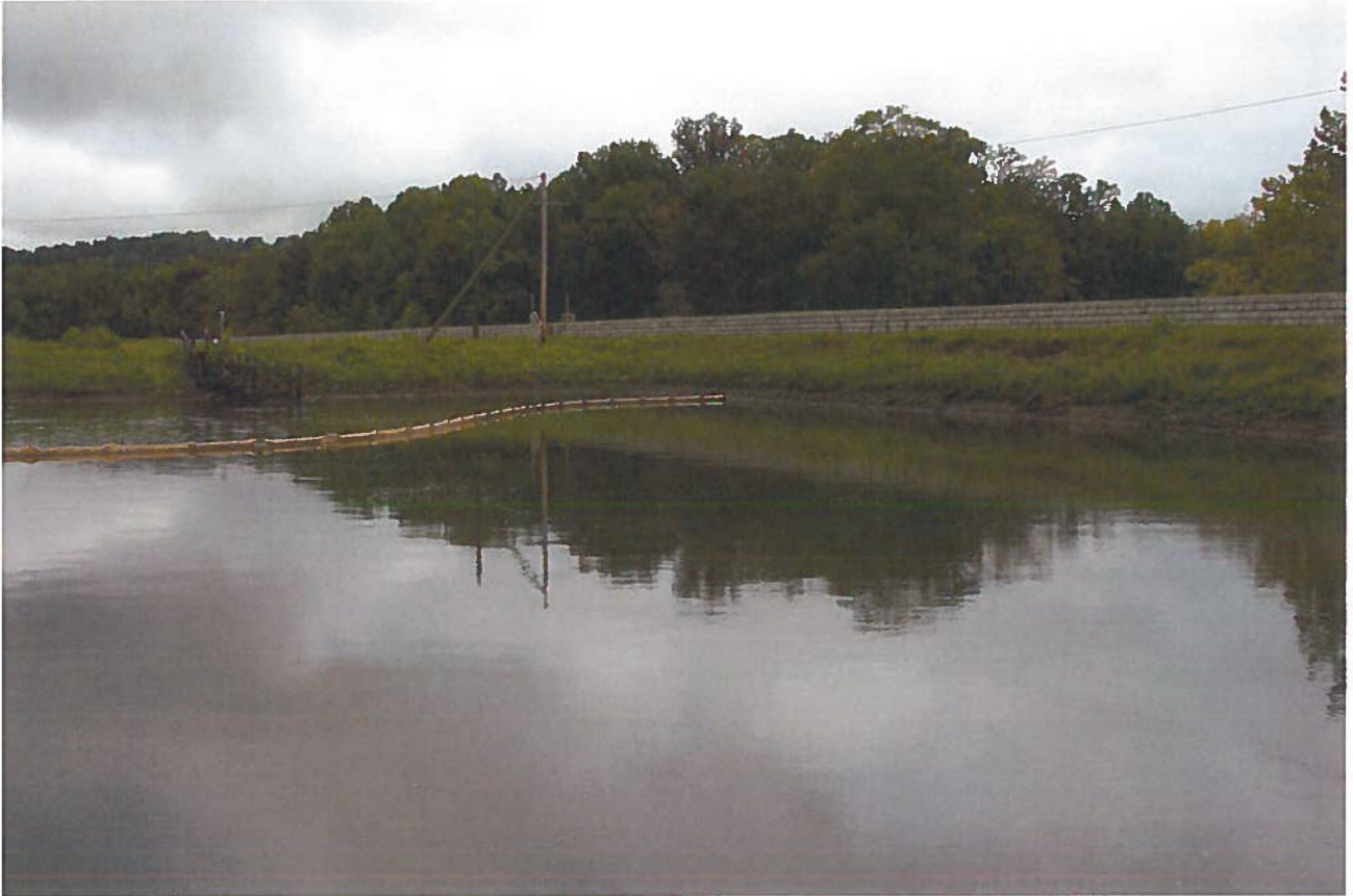
Photograph 5. Pond 1B and Upstream Slope.
