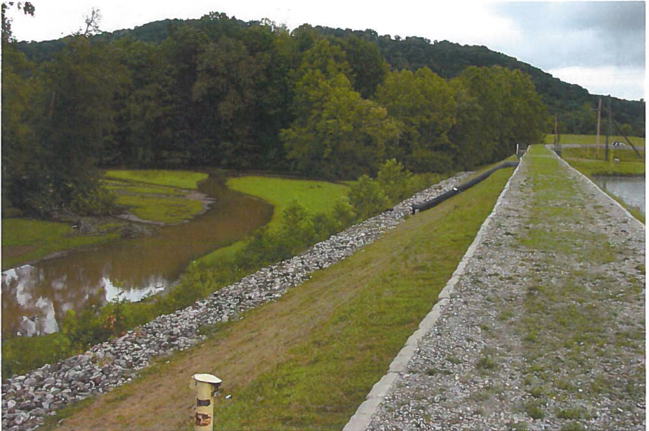
Photograph 3. Downstream Slope and Bills Creek.
