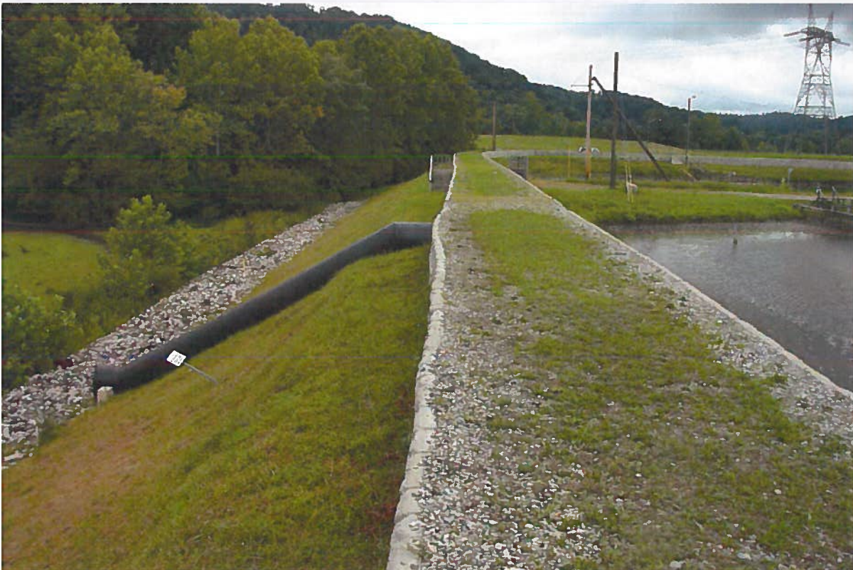
Photograph 2. Reclaim Pond Spillway Pipe and Downstream Slope.
