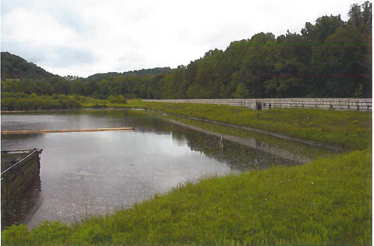
Photograph 6. Reclaim Pond and Upstream Slope.
