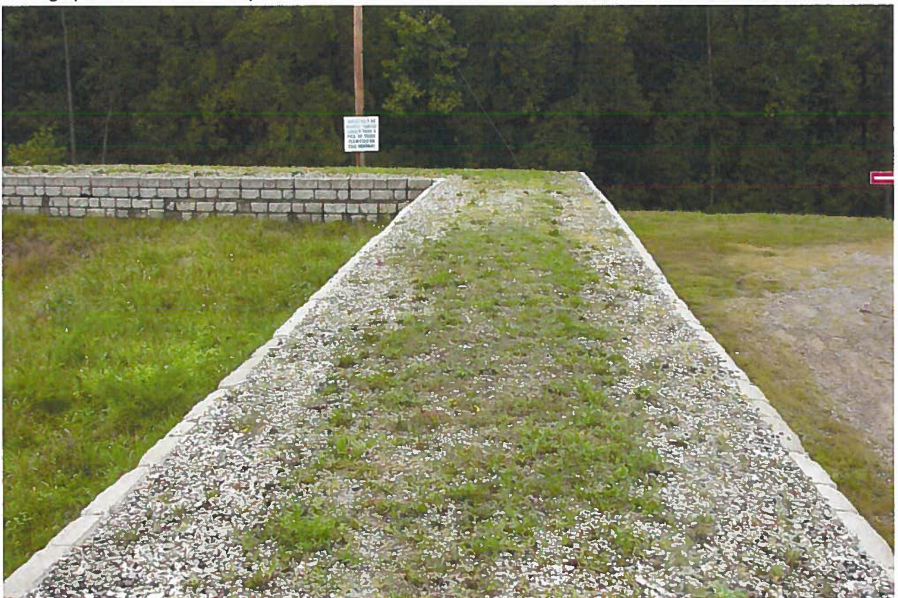
Photograph 4. Redi-rock Soil Reinforcement.
