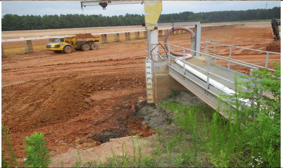
Photograph No. 11 Overflow discharge structure.
