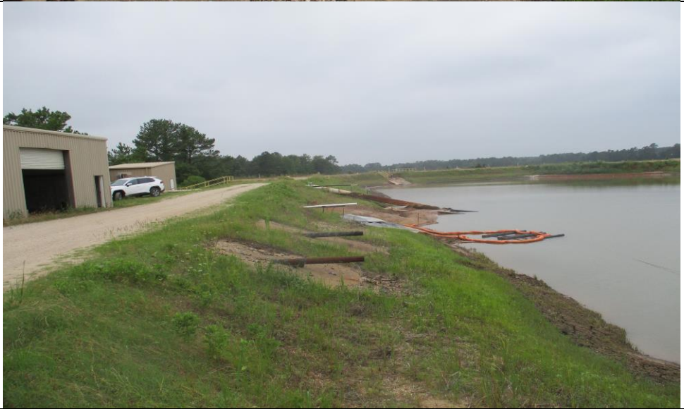
Photograph No. 20 South dike of the pond (looking west).
