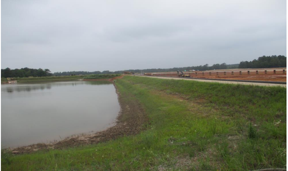
Photograph No. 22 North dike of the pond.22
