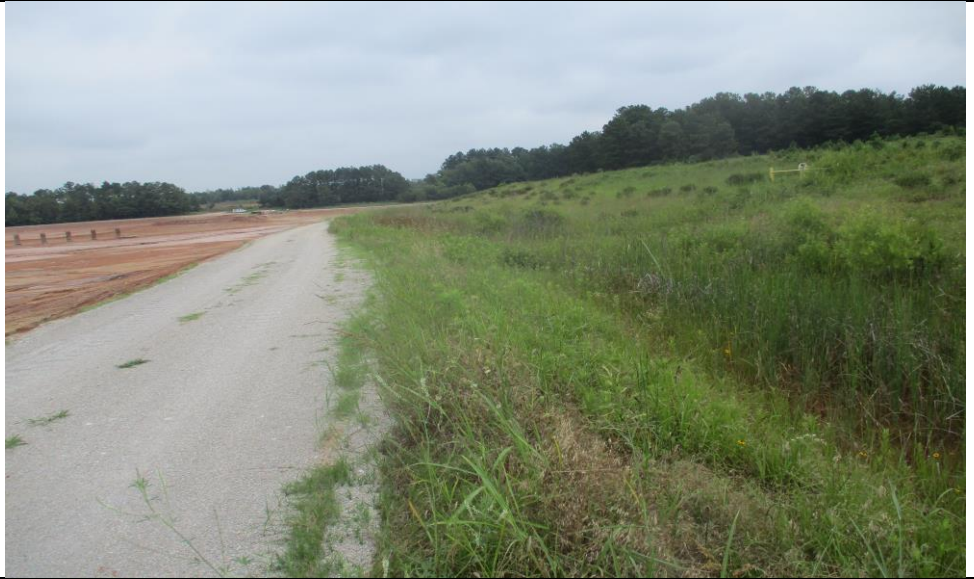
Photograph No. 6 View of the crest and toe ditch area.
