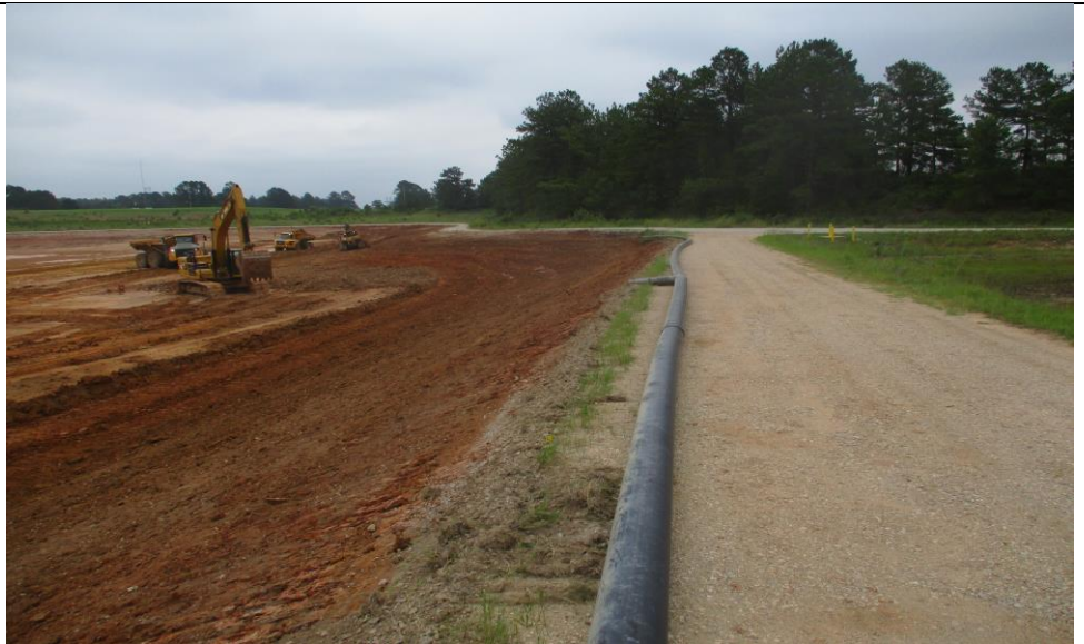
Photograph No. 1 The upstream of the south dike (looking east).
