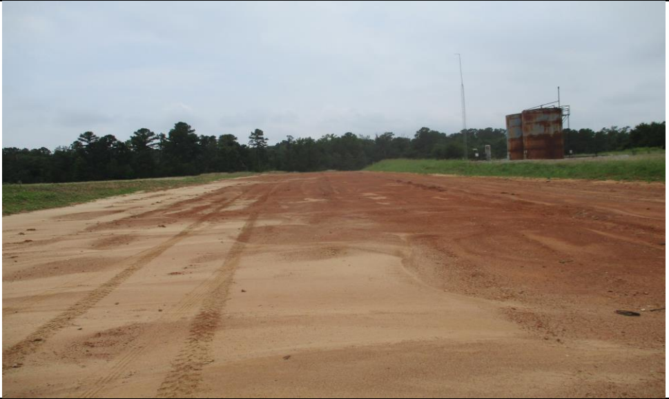
Photograph No. 17 Typical view of the west dike.
