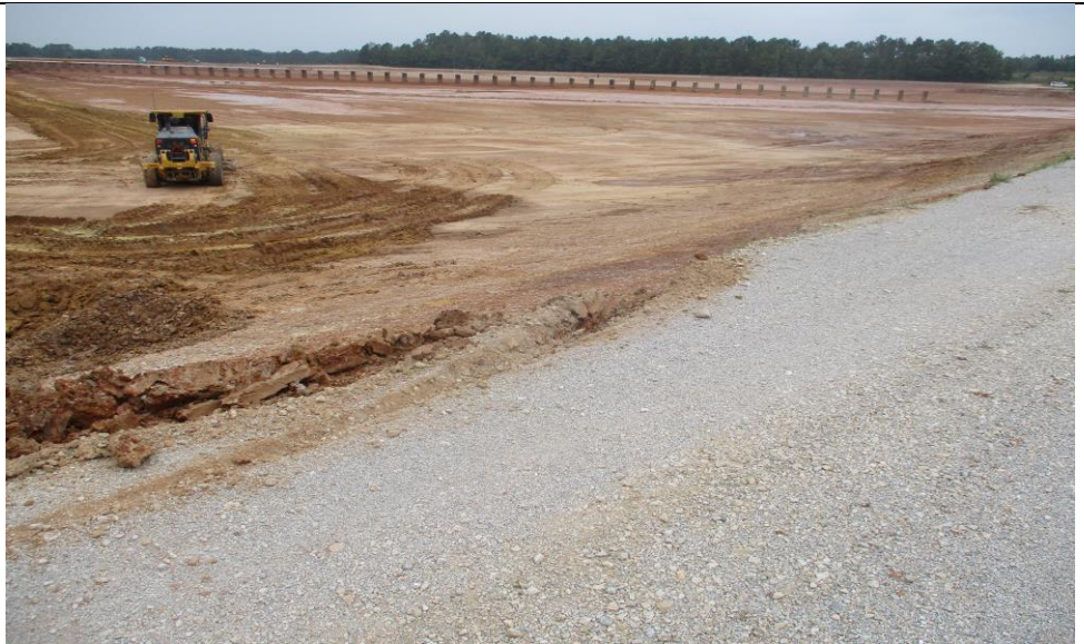
Photograph No. 7 Pond closure work in progress.
