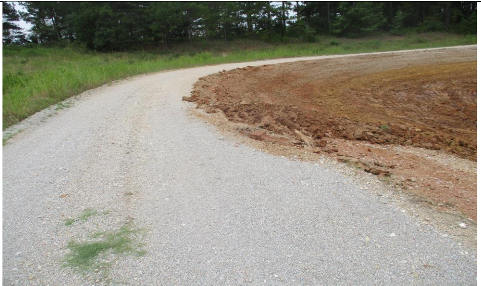
Photograph No. 4 View of typical north crest of the east pond.
