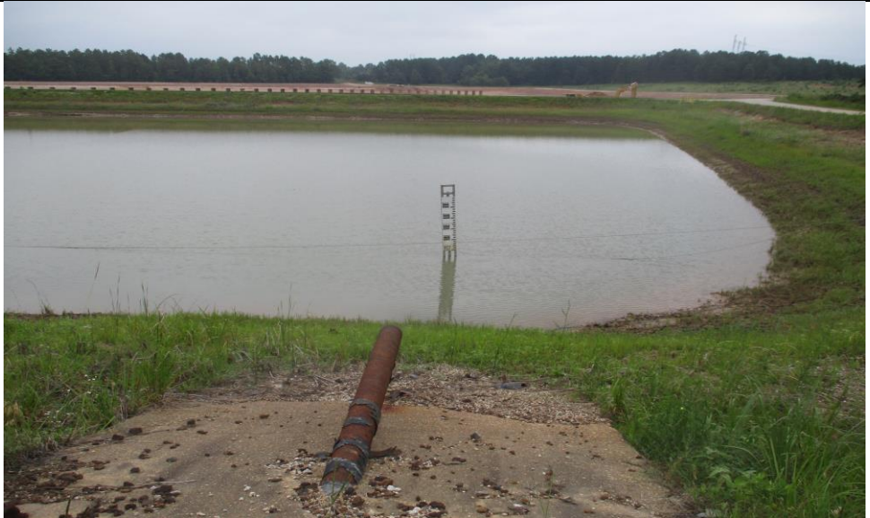
Photograph No. 19 View of the secondary bottom ash pond (looking north).
