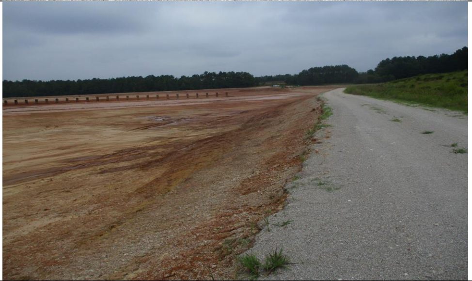
Photograph No. 5 Upstream slope and pond inside.
