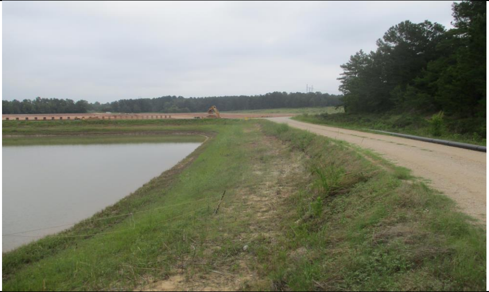
Photograph No. 21 East dike of the pond (looking north).
