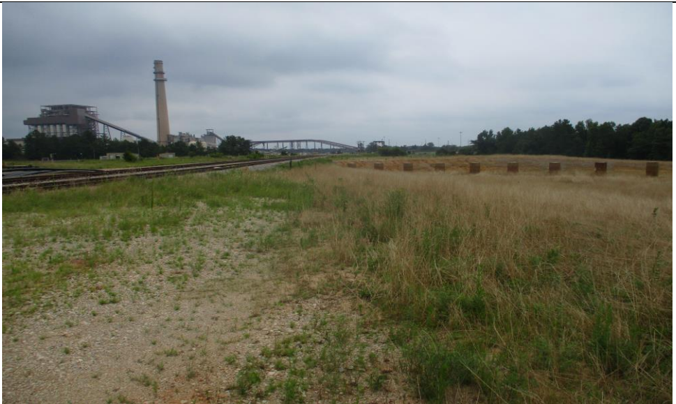
Photograph No. 15 East dike (looking south).
