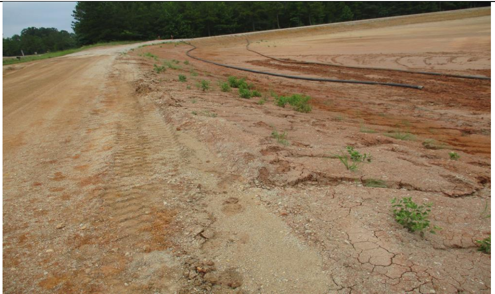
Photograph No. 10 The west dike between the ash ponds (looking north).
