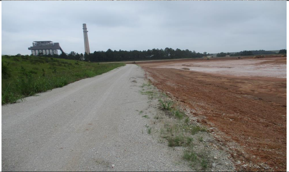
Photograph No. 8 Typical view of the crest.
