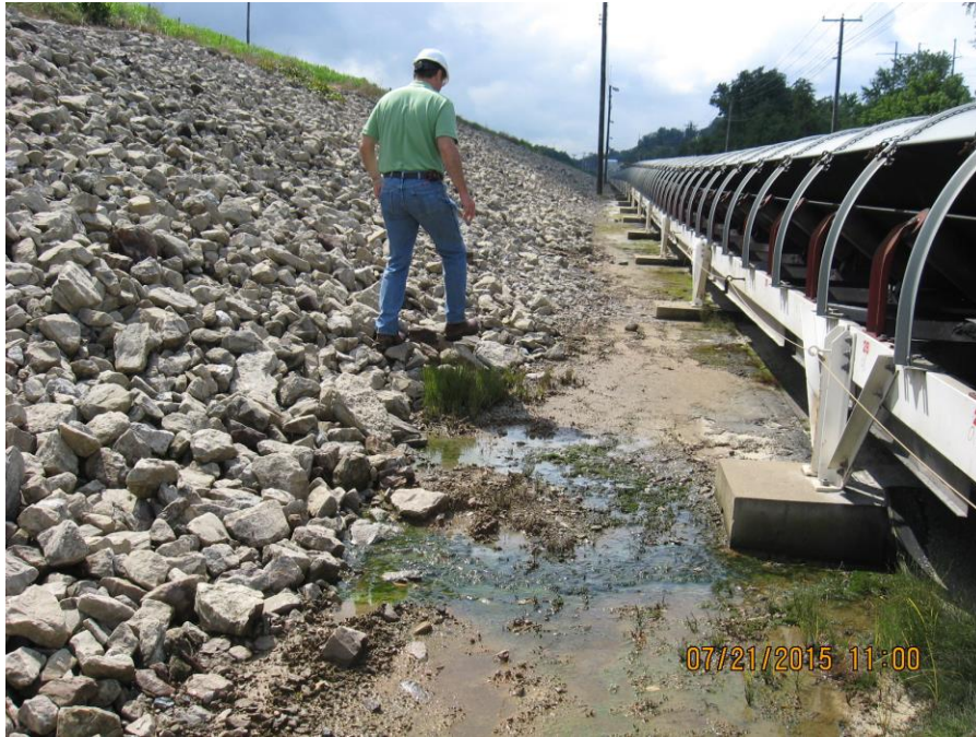
Photo 23: West Bottom Ash Pond, west dike: water near the exterior toe.
