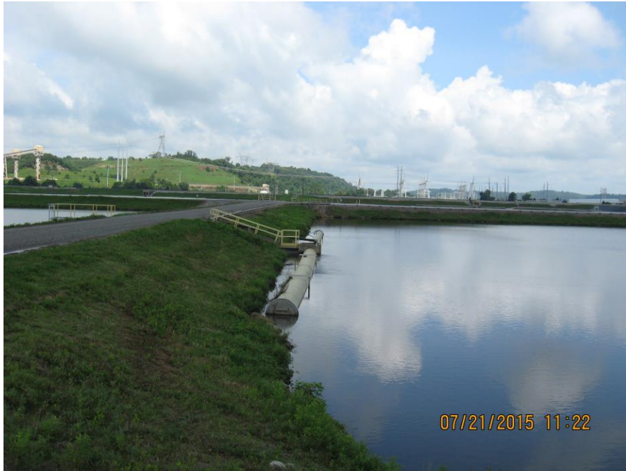
Photo 33: Clearwater Pond, west dike.
