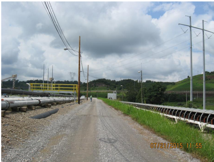
Photo 52: East Bottom Ash Pond, north dike.
