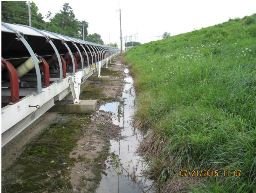
Photo 24: West Bottom Ash Pond, west dike: water near the exterior toe.
