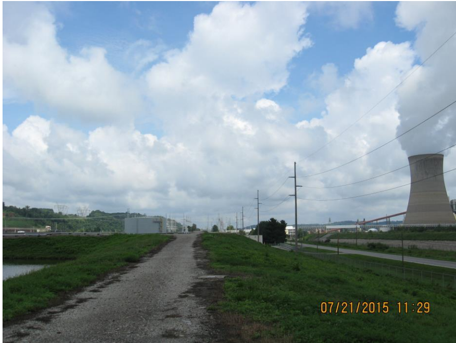
Photo 41: Clearwater Pond, east dike.
