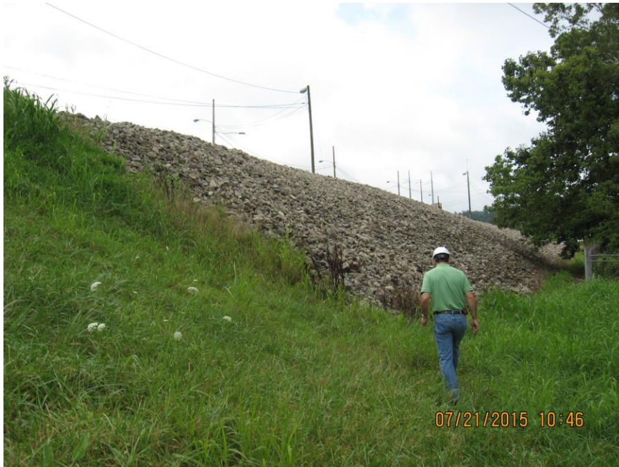
Photo 14: Bottom Ash Ponds, north dike: exterior slope.
