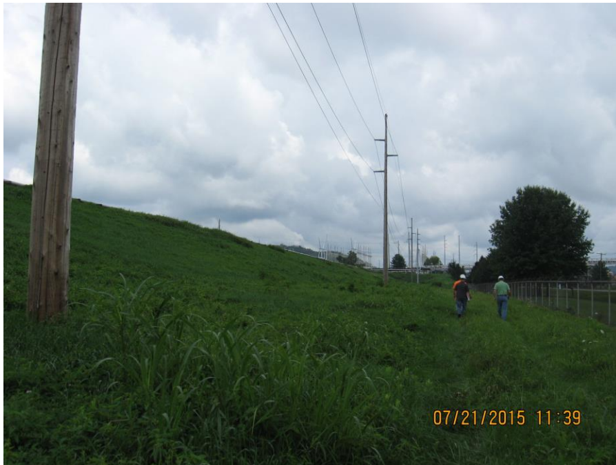
Photo 44: East Wastewater Pond, east dike.
