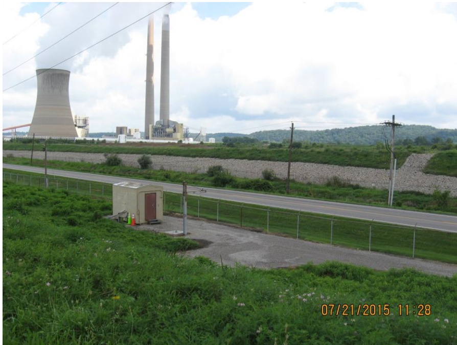
Photo 40: Clearwater Pond, east dike: exterior slope.
