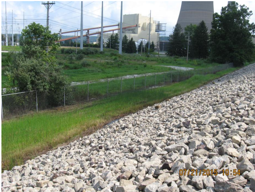
Photo 20: Bottom Ash Ponds, north dike: exterior slope.
