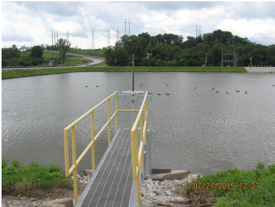
Photo 60: Clearwater Pond: outlet structure.
