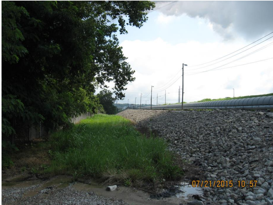
Photo 21: Bottom Ash Ponds, north dike: exterior slope.
