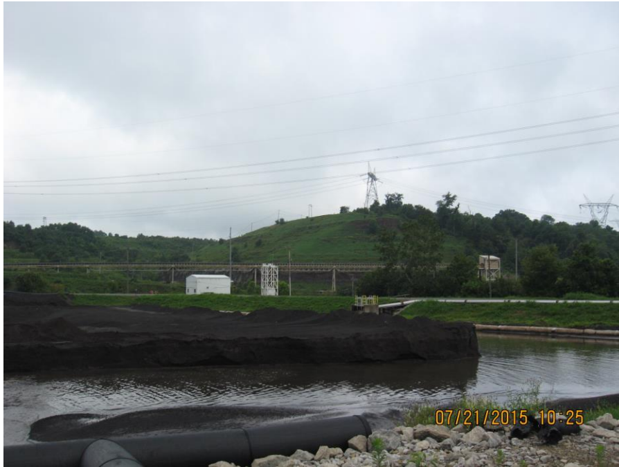
Photo 1: West Bottom Ash Pond, north dike.
