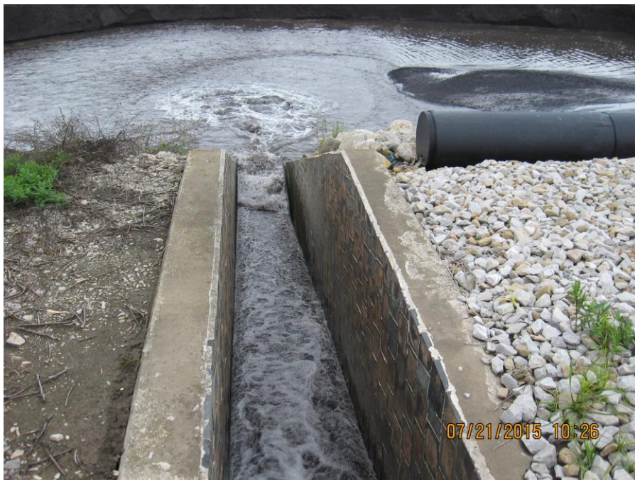
Photo 6: West Bottom Ash Pond: inlet structure.
