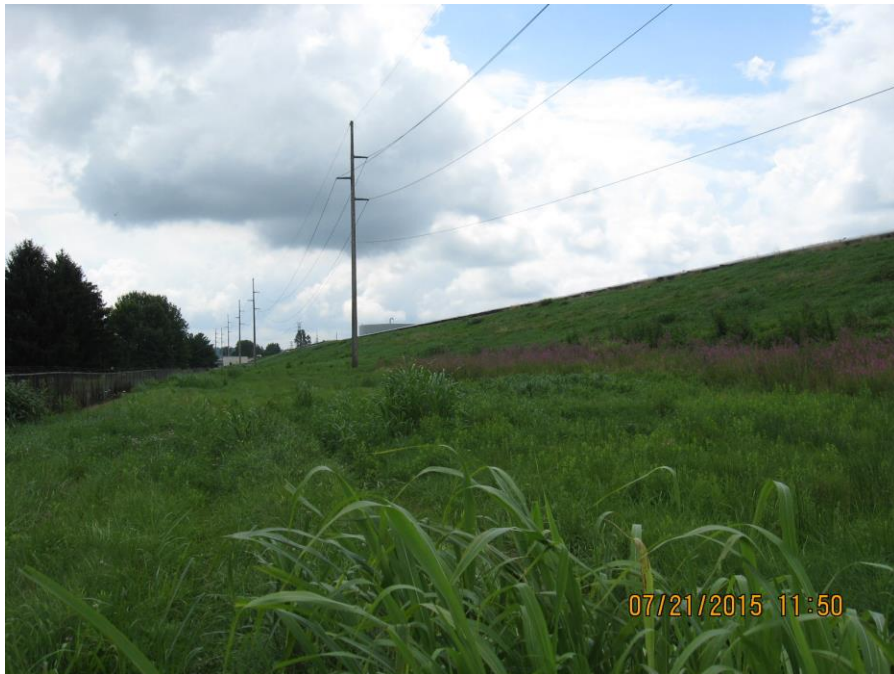
Photo 50: East Bottom Ash Pond, east dike: exterior slope.
