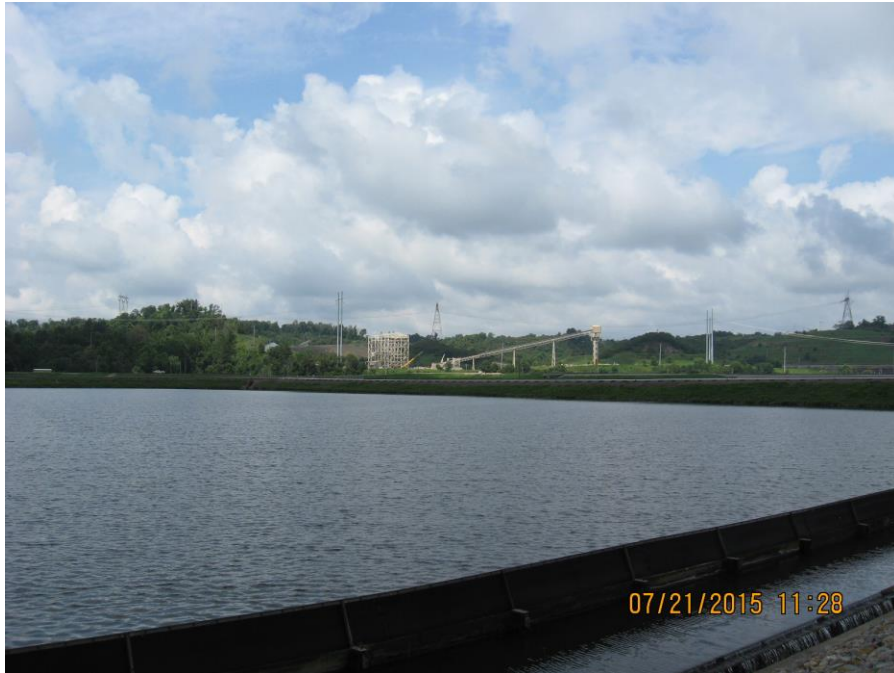
Photo 37: Clearwater Pond, north dike.
