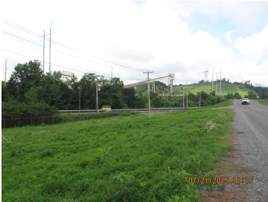
Photo 29: West Waste Water Pond, west dike.
