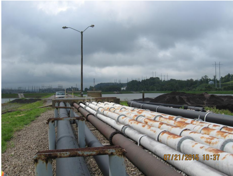
Photo 11: Bottom Ash Ponds, splitter dike: bottom ash inlet pipes.
