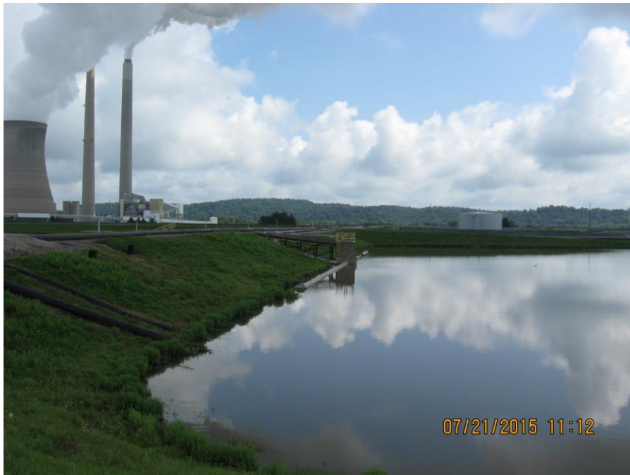
Photo 26: West Waste Water Pond, north dike.
