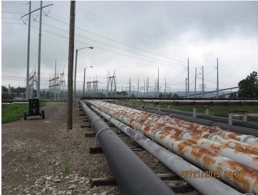
Photo 3: Bottom Ash Ponds, splitter dike: bottom ash inlet pipes.
