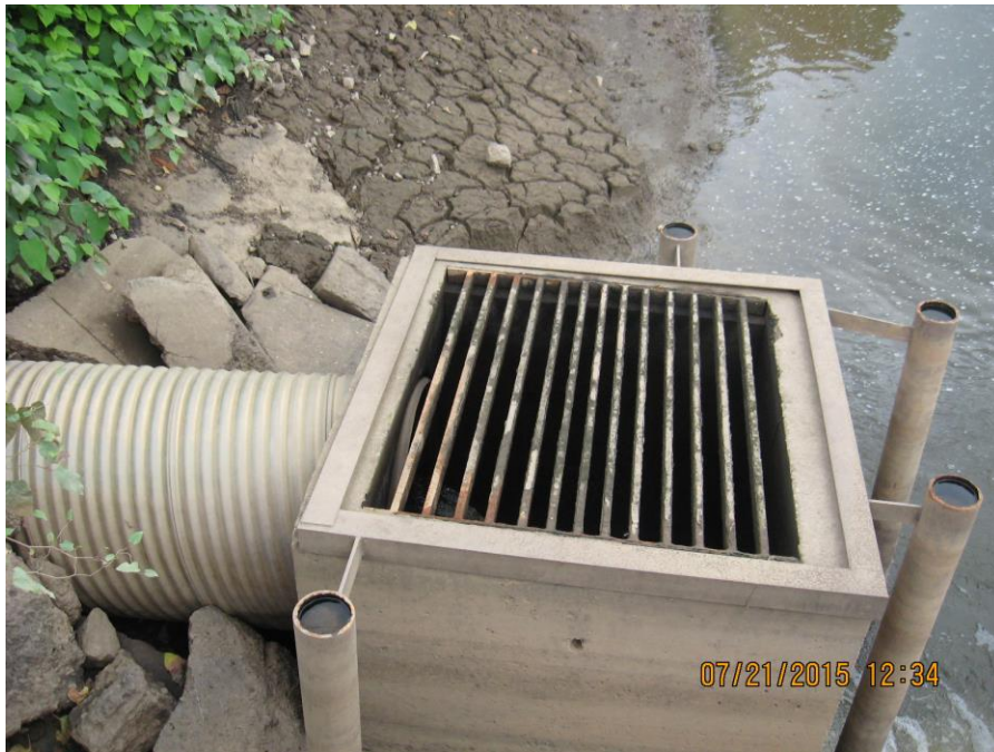
Photo 61: Ohio River outlet structure.
