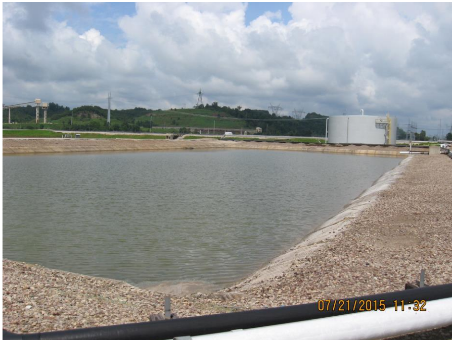
Photo 42: Leachate Surge Pond.
