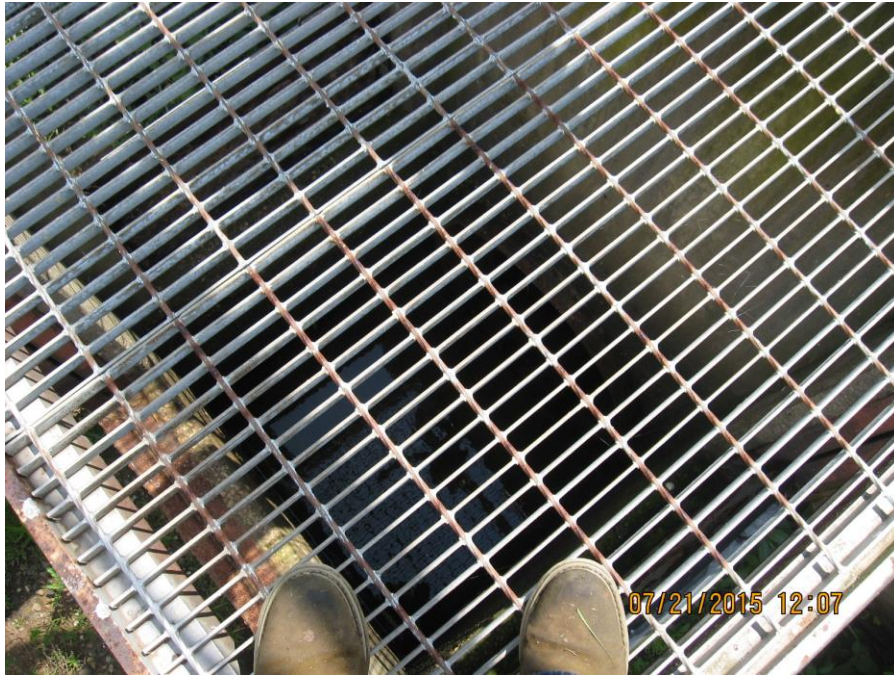
Photo 55: East Bottom Ash Pond, south dike: outlet structure.
