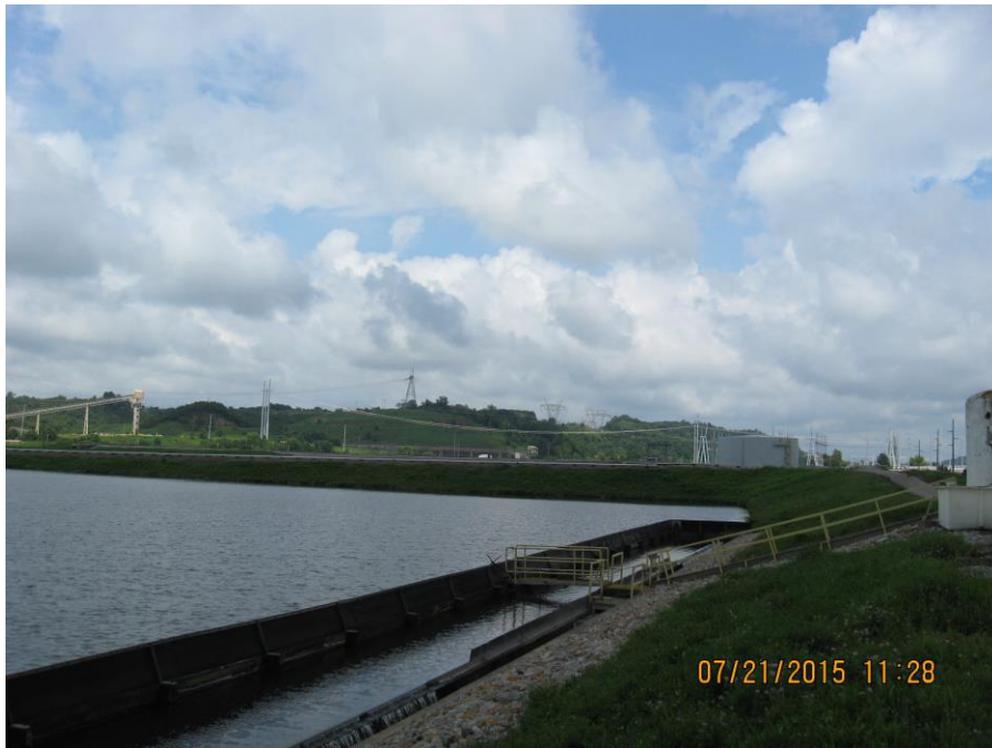
Photo 38: Clearwater Pond, east dike.
