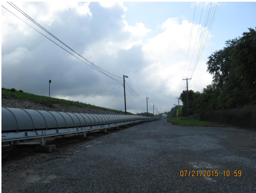
Photo 22: West Bottom Ash Pond, west dike: exterior slope.
