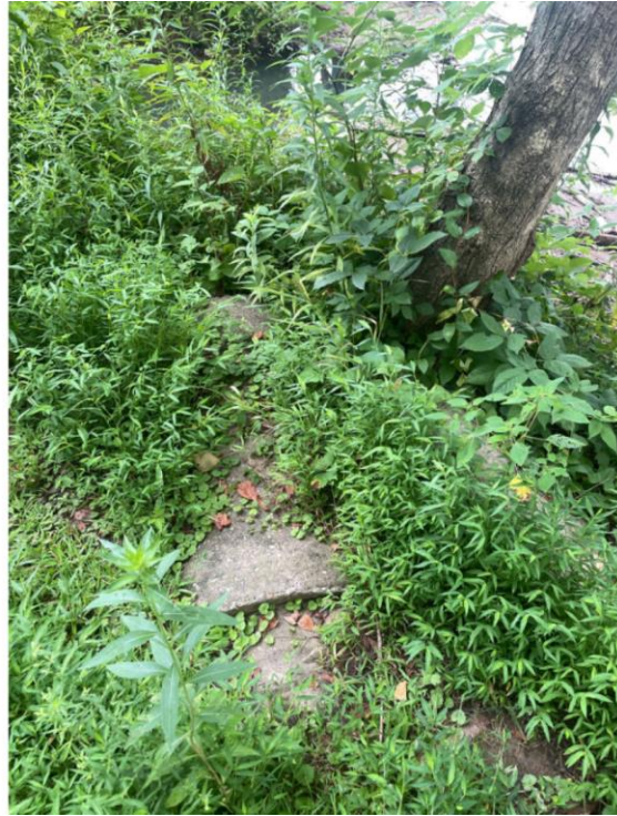
Media 28: Concrete spillway outlet pipe
