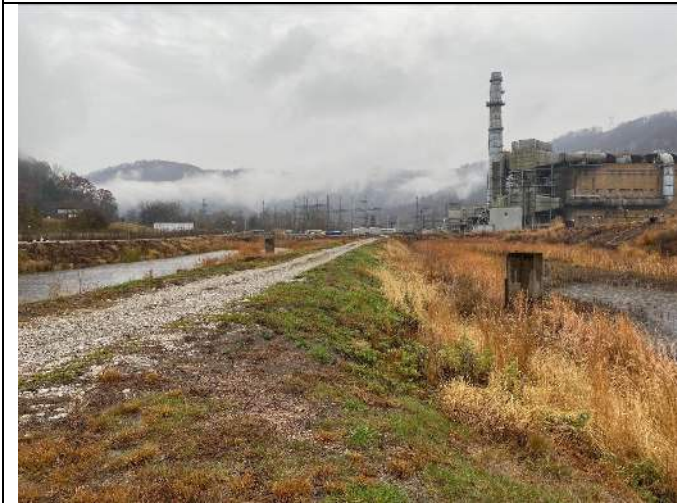
Photograph 8: View of the splitter dike separating the North and South Bottom Ash Ponds.
