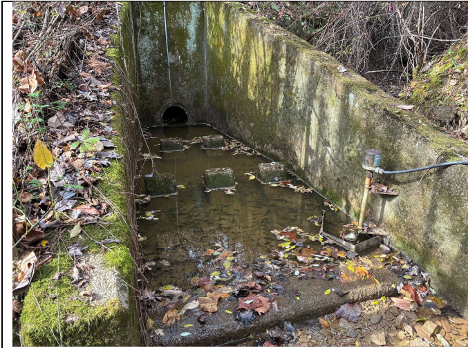
Photograph 14: Stilling basin from low flow outlet pipe.
