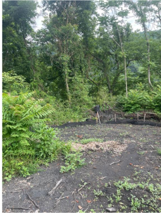
Media 36: Cleared area on the top of the ash pond with in-place erosion control measures (recently cleared)
