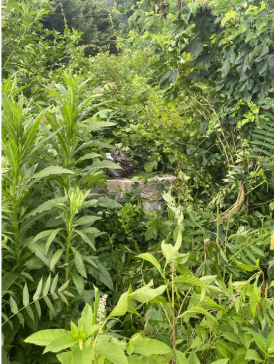
Media 43: Top of concrete stormwater manhole. Access point for stormwater drainage pipes that traverse the ash pond
