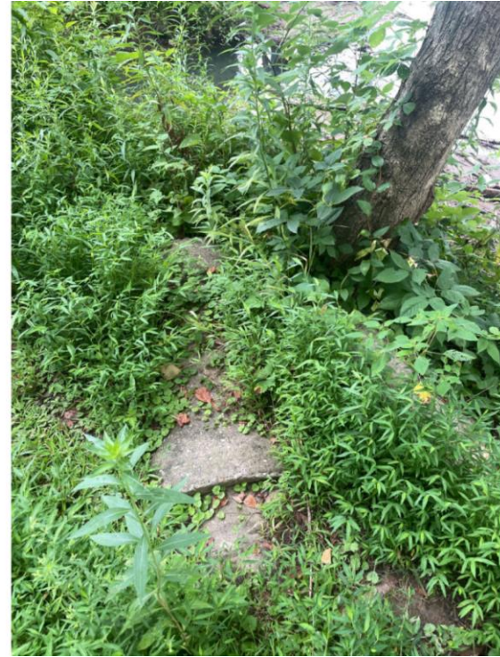
Media 28: Concrete spillway outlet pipe
