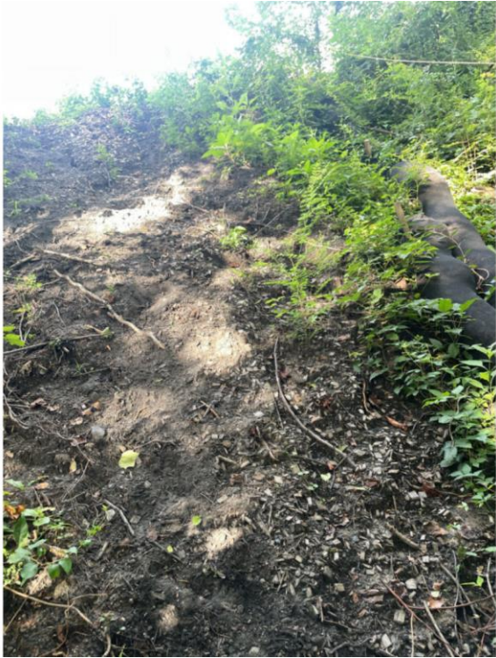
Media 9: Erosion control measures on perimeter dike
