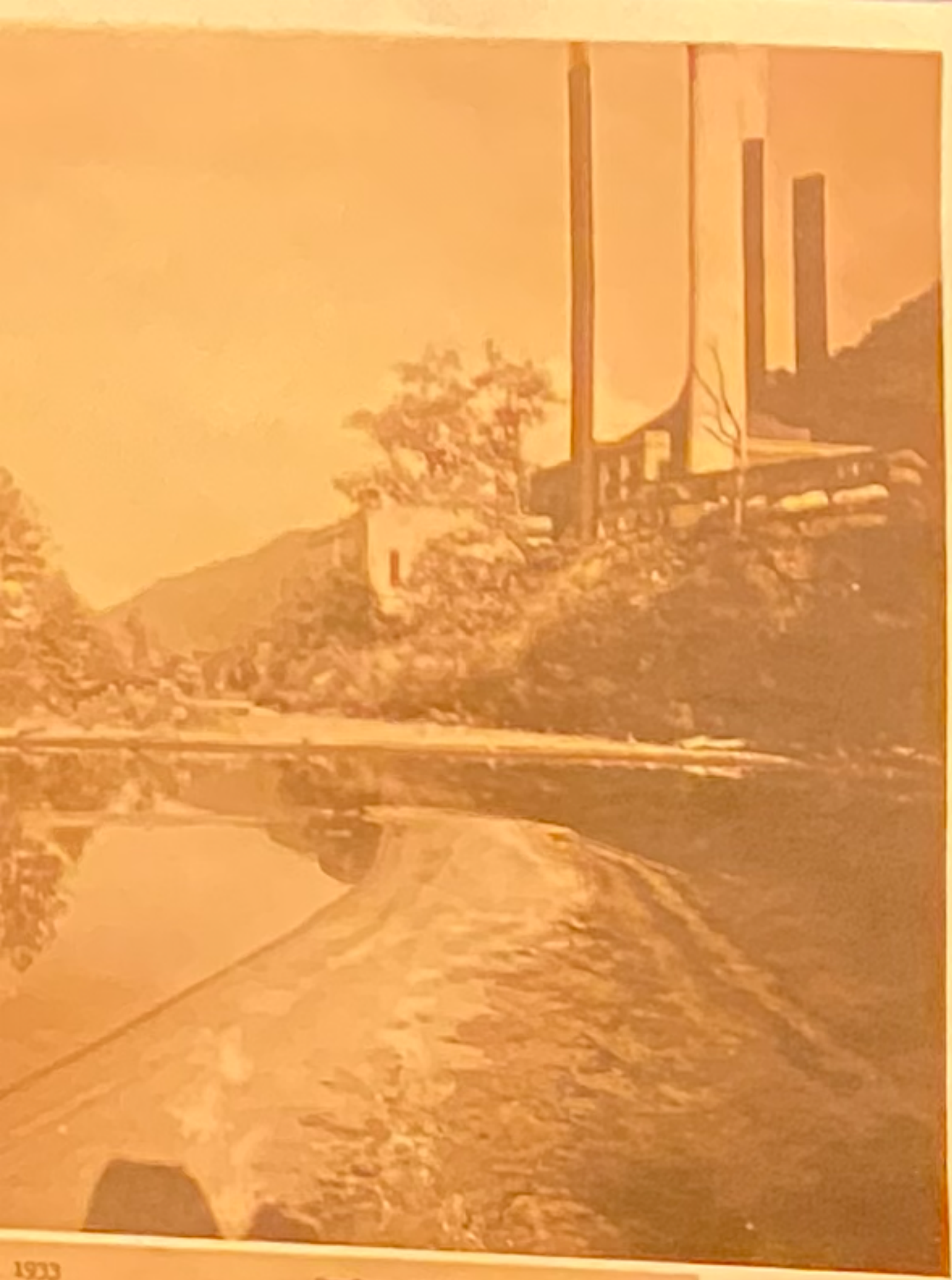
1933 Surface of Reser Elevation 579.2 Normal Pool Elevation 577.9 View upstream along left bank of Kanawha River from as shown at the mouth of Cabin Creek
