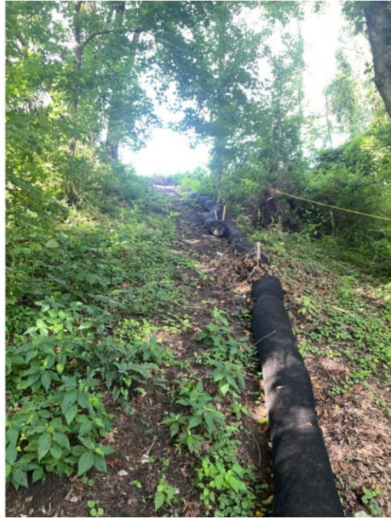
Media 8: Erosion control measures on perimeter dike
