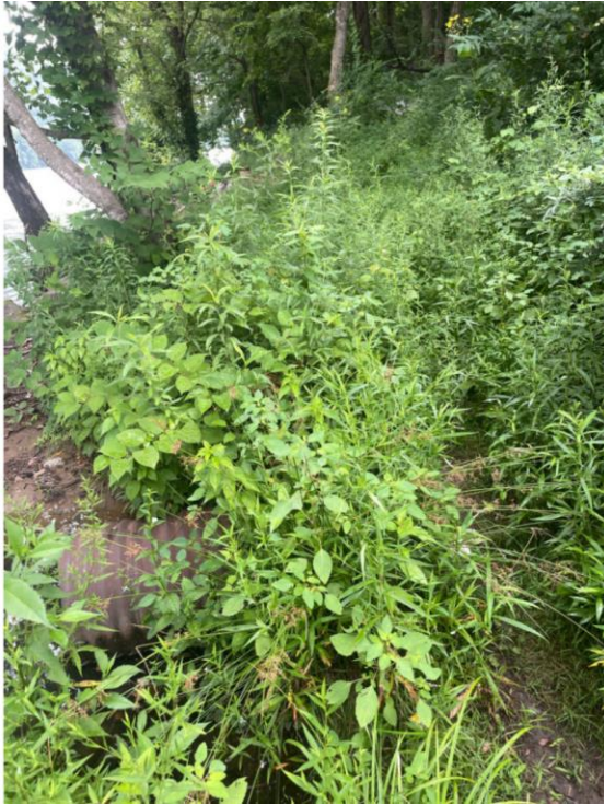
Media 27: Corrugated metal storm water pipe by the concrete outlet pipe
