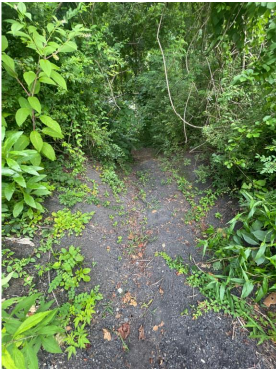
Media 33: Perimeter dike at the northwest end of the ash pond
