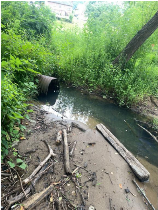
Media 29: Corrugated metal storm drain outlet
