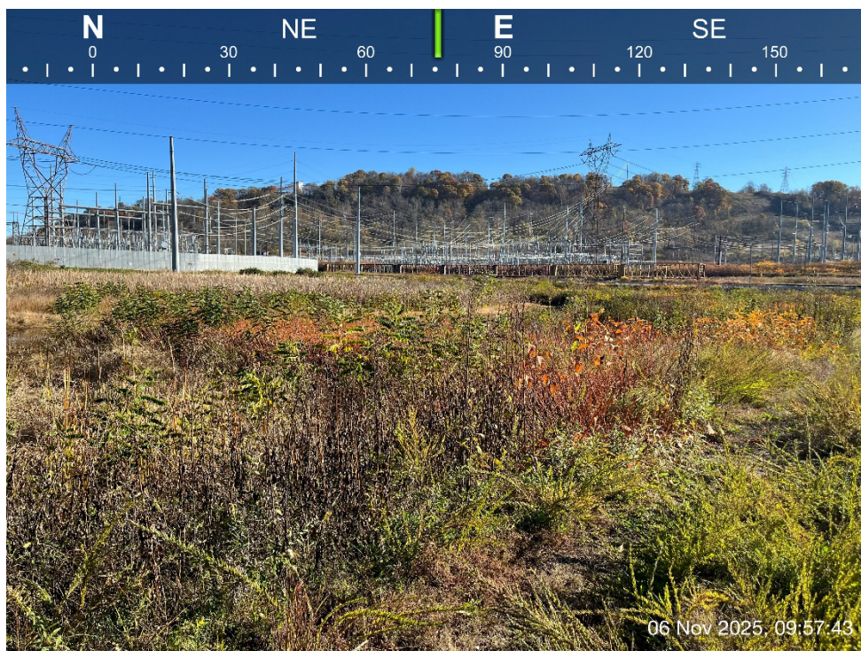
Photograph 6. View of Kammer 345 kV Station.
