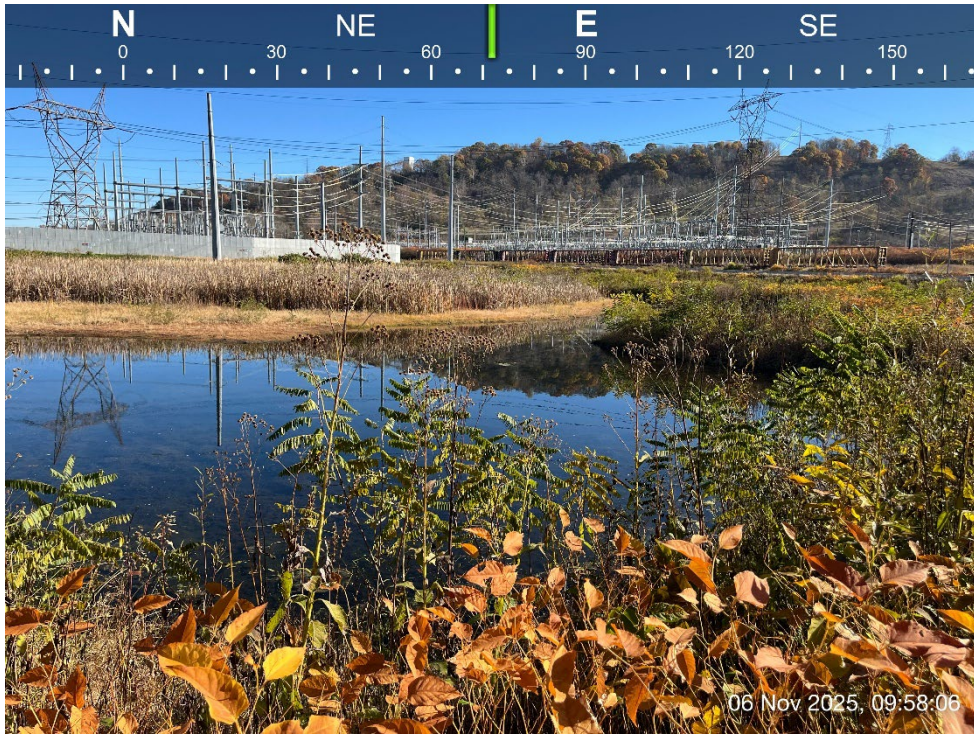
Photograph 7. View of northern section of ash pond.
