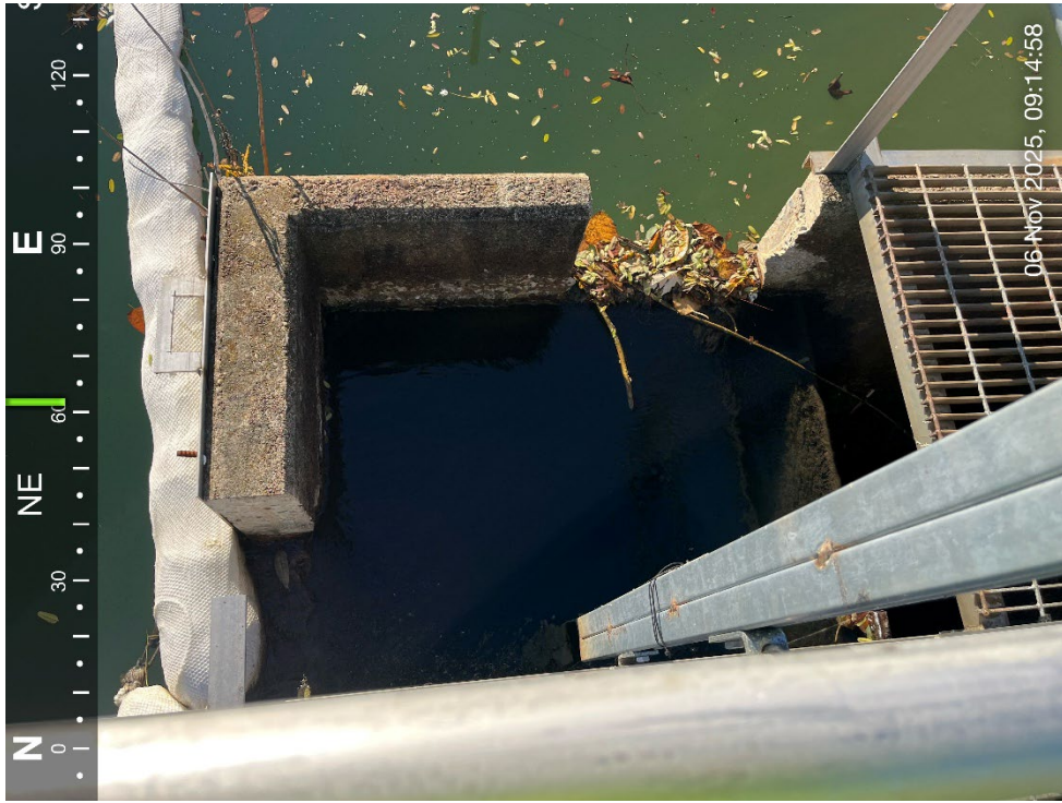
Photograph 1. Ash pond outlet control structure.
