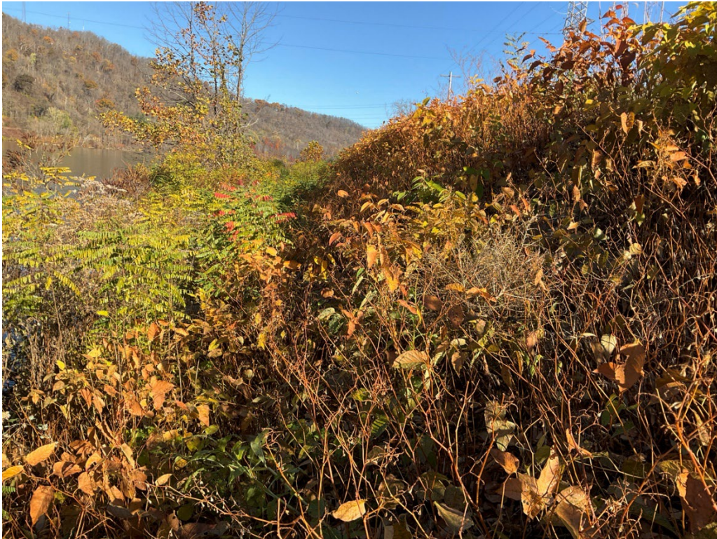
Photograph 3: View of the exterior dike slope looking north.
