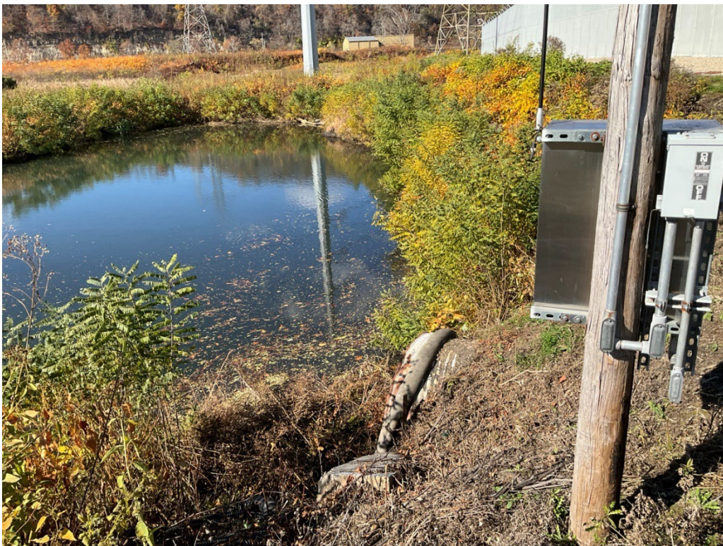
Photograph 8: View of 60-inch diameter CMP outlet at northeast corner of Ash Pond.
