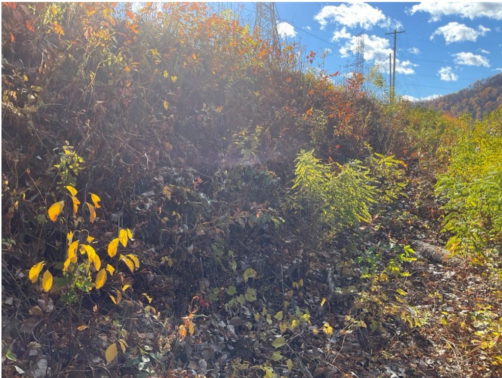
Photograph 6: View of the exterior dike slope looking south.
