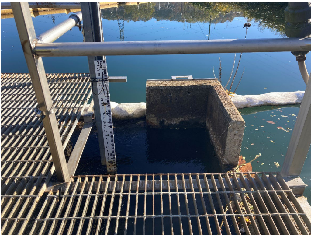
Photograph 12: View of the spillway concrete weir notches looking east.
