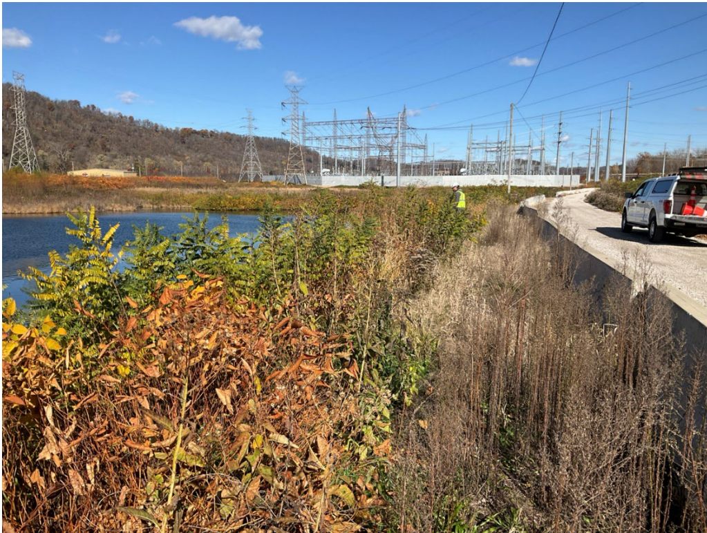
Photograph 10: View of the interior dike slope looking north.
