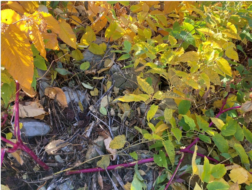
Photograph 14: View of rip rap along exterior dike slope.
