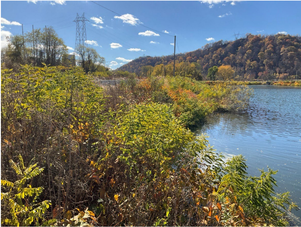
Photograph 9: View of the interior dike slope looking south.
