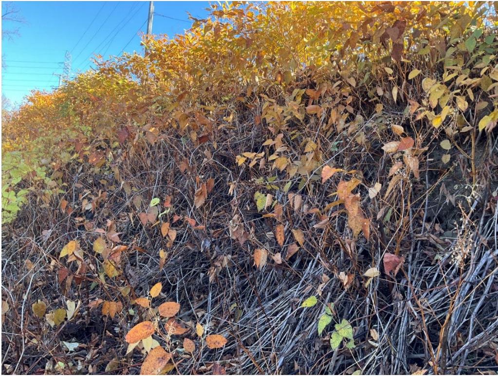
Photograph 5: View of the exterior dike slope looking north.
