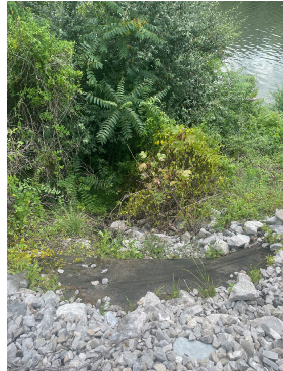
Media 8: Southern slope of EFA showing erosion damage on perimeter dike adjacent to the Kanawha River
