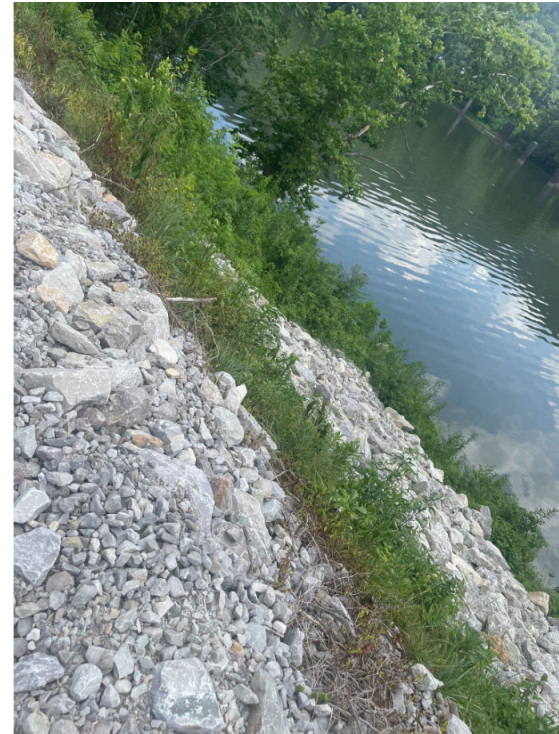
Media 12: Southern slope of EFA along the Kanawha River showing erosion repair that was backfilled with geotextile and riprap
