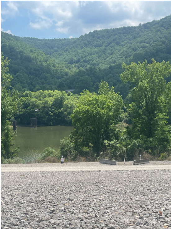
Media 17: Top of EFA cover looking south towards the Kanawha River. Showing surge stone on top of the geosynthetic cover system
