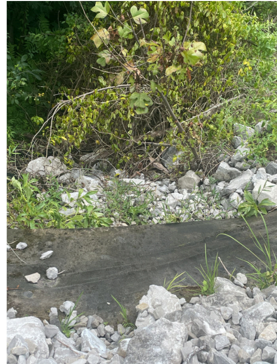
Media 6: Southern slope of EFA looking towards the Kanawha River. Showing erosion repairs on steeper dike slopes
