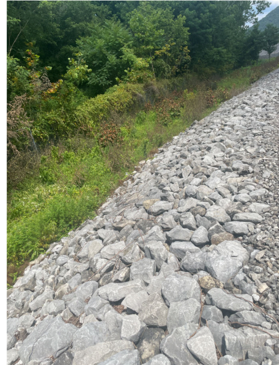
Media 4: Northern slope of EFA looking west shows riprap armoring on slope
