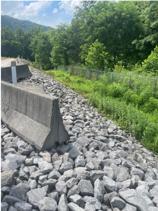
Media 5: Northern slope of the EFA looking west. Showing riprap armoring on the slope
