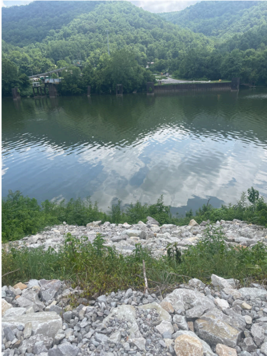
Media 13: Southern slope of EFA along the Kanawha River showing erosion repair that was backfilled with geotextile and riprap
