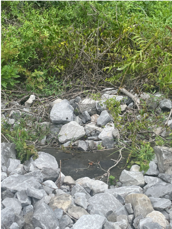
Media 7: Southern slope of EFA looking towards the Kanawha River showing riprap repair section on dike and soil/vegetative slope below
