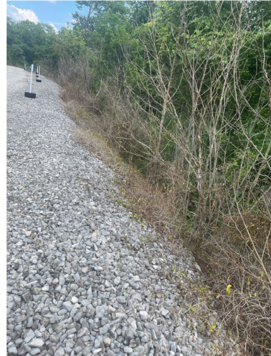
Media 16: Southern slope of EFA along dike crest showing stone base for access road and heavily vegetated area on slope
