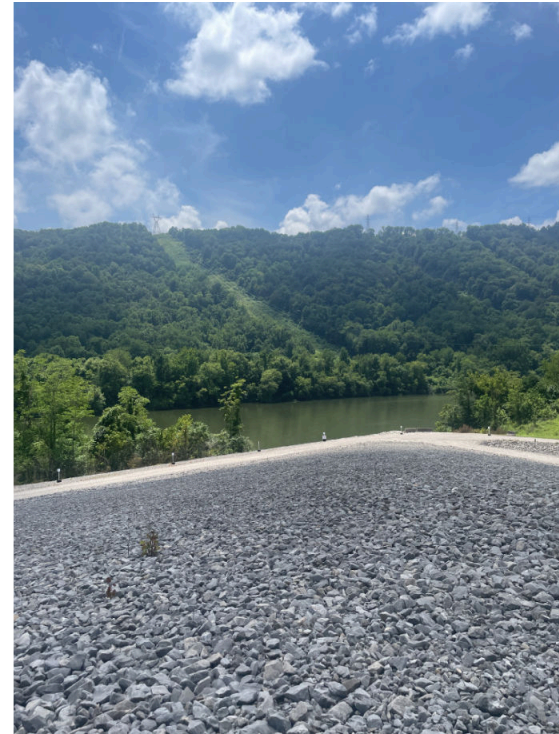
Media 18: Top of EFA looking southwest towards the Kanawha River (surge stone cover material)
