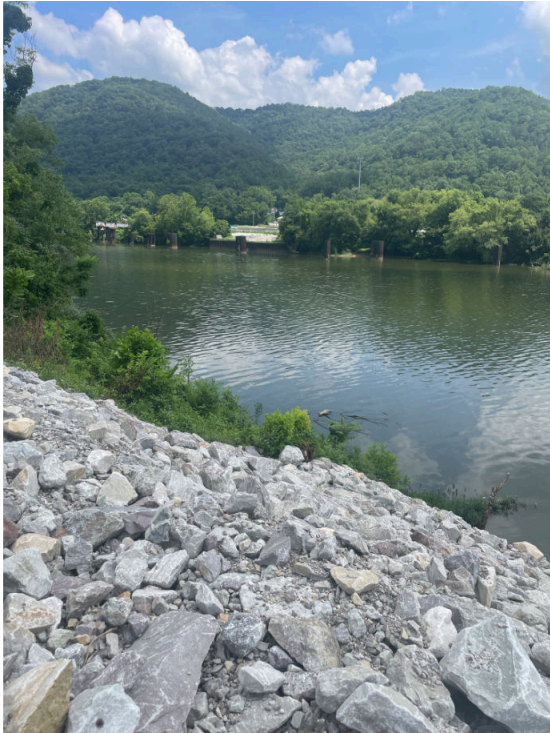
Media 9: Southern slope of EFA showing repaired erosion area along the Kanawha River
