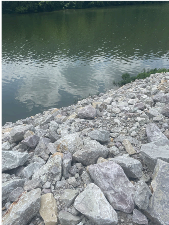
Media 11: Southern slope of EFA showing repaired erosion area along the Kanawha River. Repairs extend to the water level
