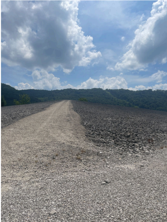
Media 3: existing stone riprap cover and path towards the eastern portion of EFA
