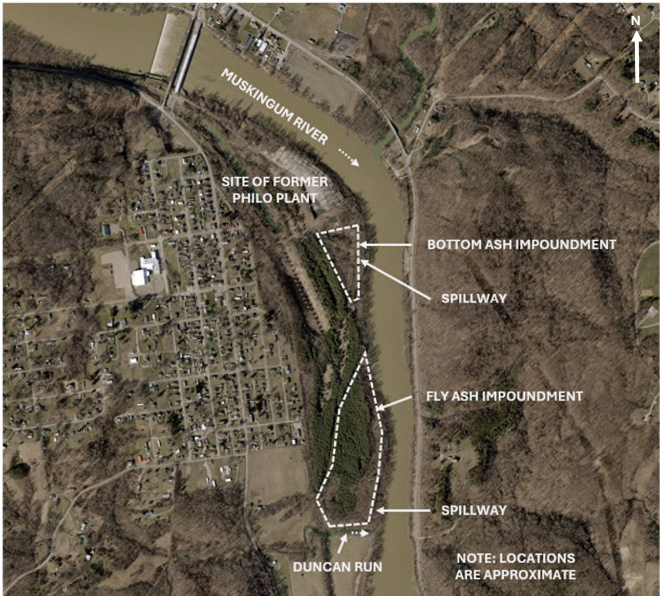
Figure 1-1 – Former Philo Plant (2020 OGRIP Image)
