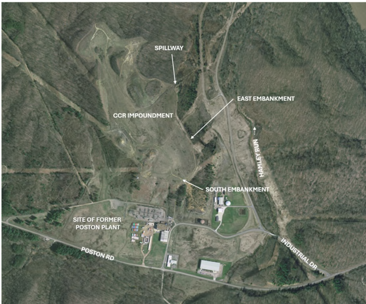
Figure 1-1 – Former Poston Plant
