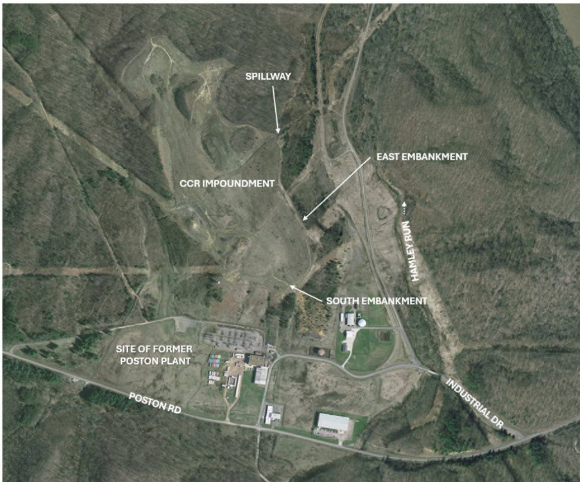
Figure 1-1 – Former Poston Plant
