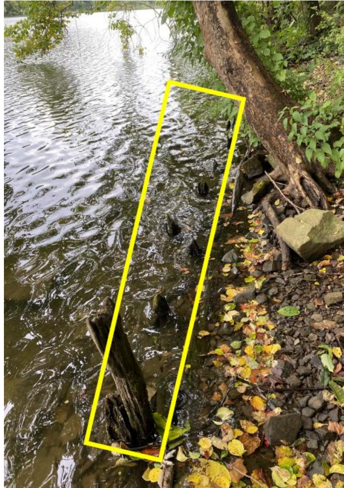
Figure 1-3: Photograph of the piles supplied prior to the WRD inspection.
