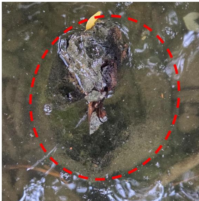
Figure 3-3: Plan view photograph of Pile 16 of Subzone B2 showing the shoulder of the pile at ground level.
