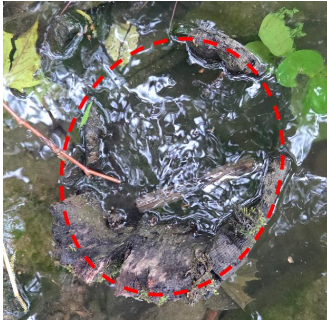
Figure 3-2: Plan view photograph of Pile 6 of Subzone B2 with only the sapwood remaining above water.
