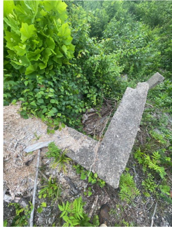
Media 34: Remnants of old concrete outlet structure used when the ash pond was active
