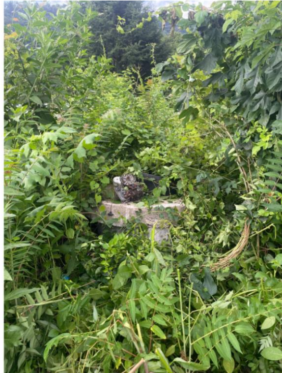
Media 42: Top of concrete stormwater manhole. Access point for stormwater drainage pipes that traverse the ash pond
